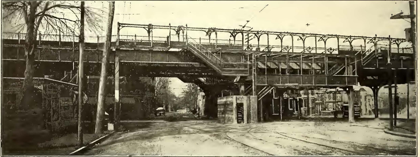
Forest Hills Extension, Boston Elevated Railway—General View of Eggleston Square Station from Columbus Avenue
