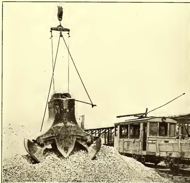
Grab Bucket Used at the Windermere Storage Yard
