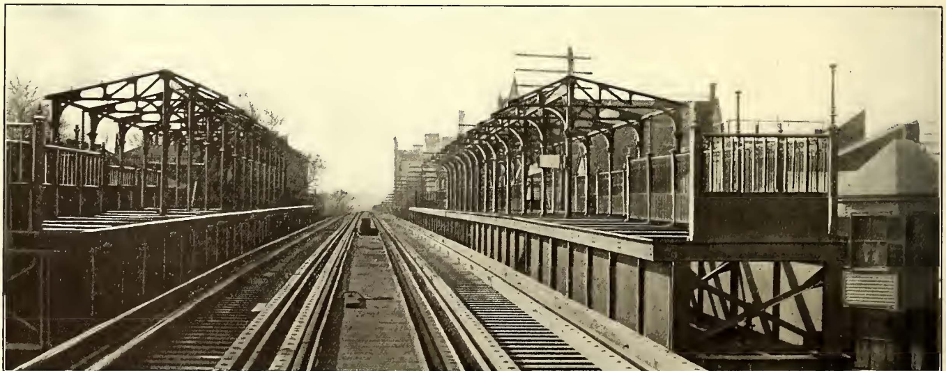
Forest Hills Extension of the Boston Elevated Railway—View of Both Platforms at Eggleston Square Station Under Construction
