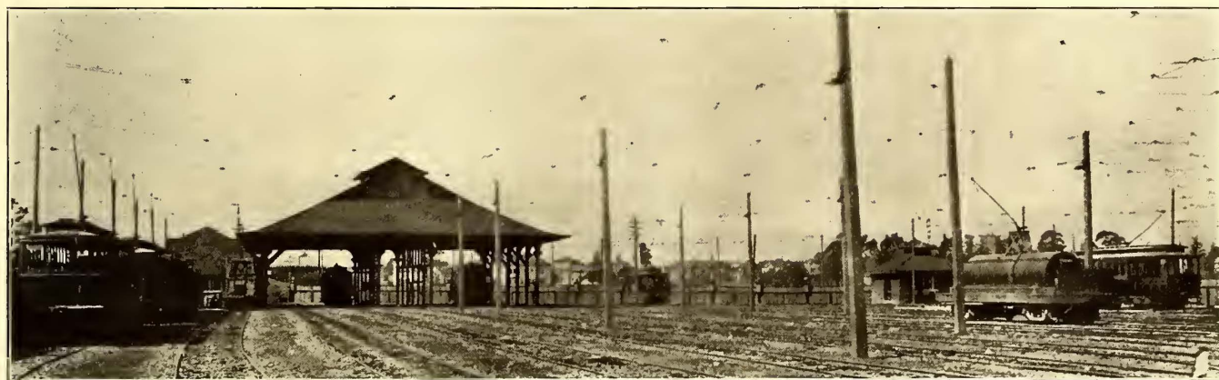
Oakland Traction Company—View of Yards and Inspection Shed
