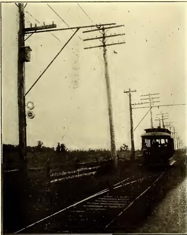
Pole Carrying Signal Box and Disks
