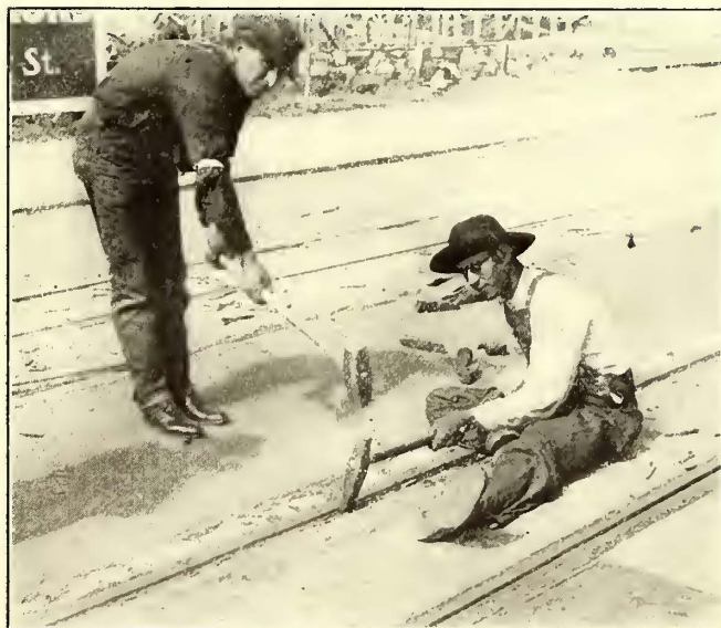
San Francisco Street Railways—Shearing Rails on McAllister Street
