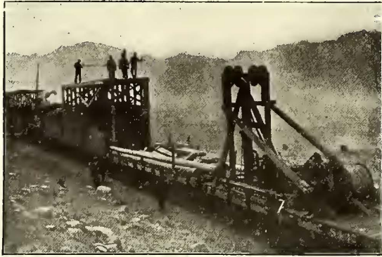
Denver & Interurban Railway—Apparatus for Stringing Wires
