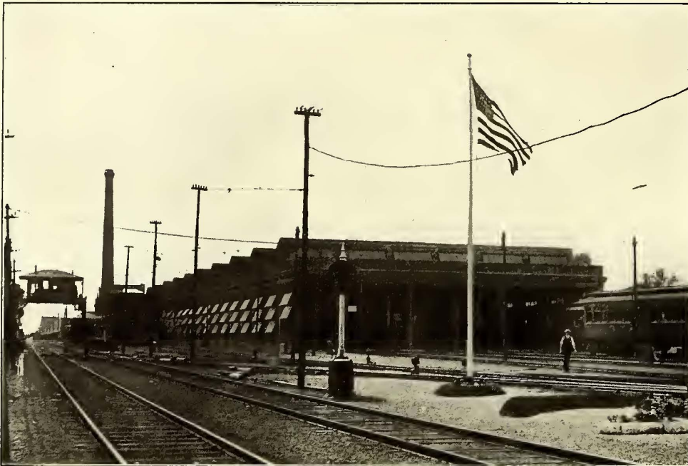
Brooklyn Shop Gardens—Front of Fresh Pond Inspection Plant
