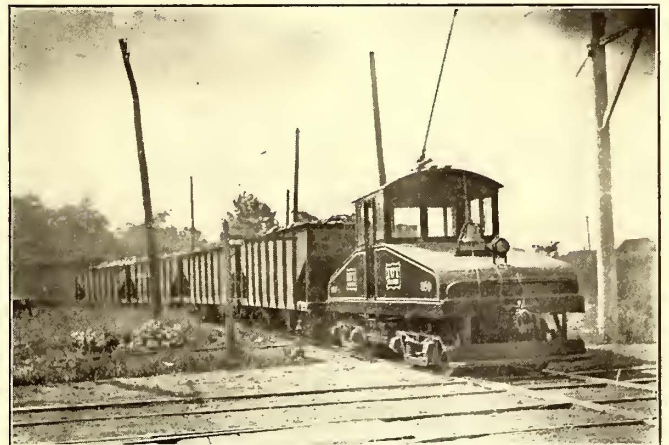
Locomotive Hauling Train of Freight Cars
