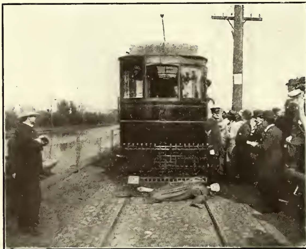
Public Service Commission Fender Tests at Schenectady—Partly Successful Pick-up of a 120-lb Dummy Placed on Cobblestone Section
