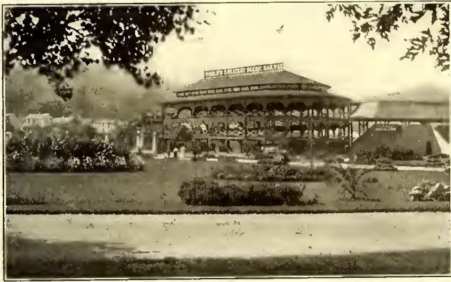
Ohio Valley Scenic Route—Scenic Railway Building in Rock Springs Park
