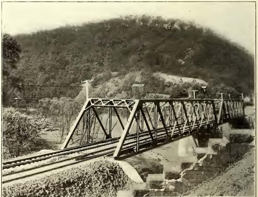
Ohio Valley Scenic Route—Bridge over Little Beaver Creek, near East Liverpool, Ohio
