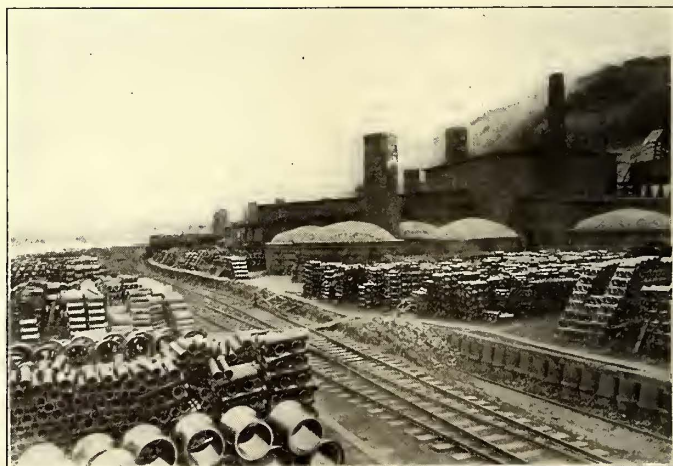
Ohio Valley Scenic Route—Sewer Pipe Works on Line of Electric Railway
