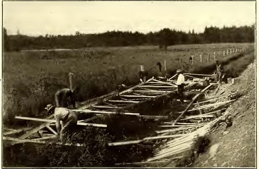
Milwaukee Transmission Line—Assembling Tower
