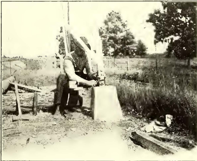
Milwaukee Transmission Line—Tower-Raising Hinge
