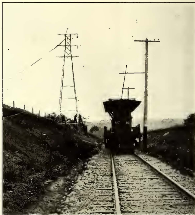
Milwaukee Transmission Line—Electric Work Car Raising Tower
