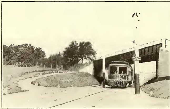
Milwaukee Transmission Line—Road Gardening
