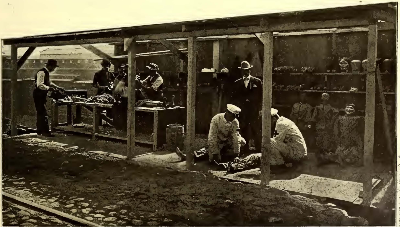
Dummy Repair Shop Built for the Schenectady Fender and Wheel-Guard Trials
