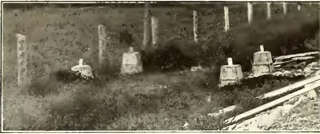
Milwaukee Transmission Line—Special Footings with Anchors
