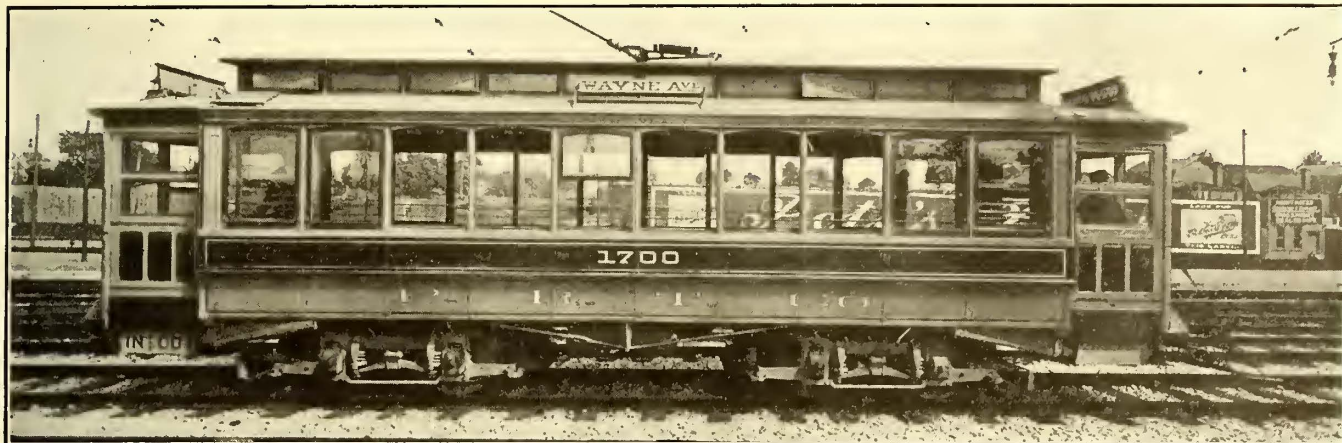
Fig. 5—Philadelphia's Pay-Within Car. Appearance of the Car When Running, Showing Both Doors Closed and the Steps Raised
