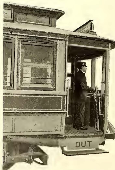
Fig. 3—Philadelphia's Pay-Within Car. Front Platform with Door Opened by Motorman for Alighting Passengers
