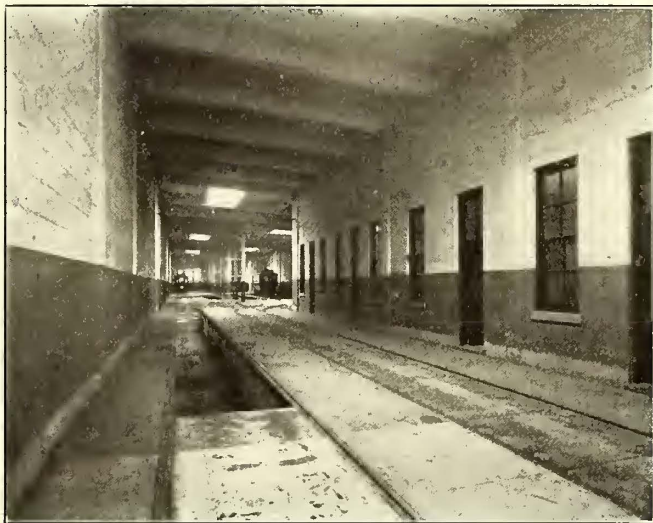
Car Houses in Baltimore—One of the Bays in the York Road Car House, Showing Track Construction Required Owing to Facilities Room at Entrance
