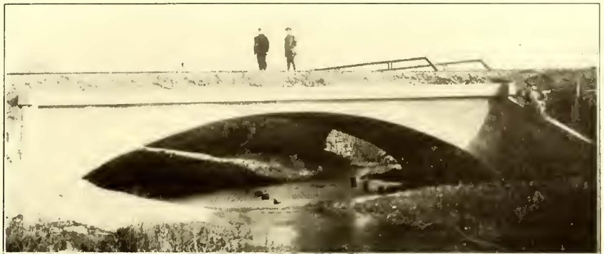
Fig. 5.—Bridge Reconstruction on the Columbus & Lake Michigan Railway—Bridge 943 of 50-ft. Span
