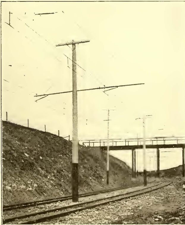
Milwaukee Interurban Lines—Catenary Construction on Curves
