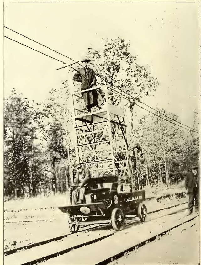
Auto Line Patrol Car—Inspecting Trolley Wire
