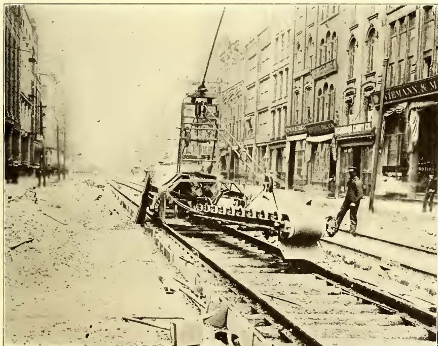
Fig. 29—Motor-Driven Concrete Mixer with Swinging Delivery Spout Used in Milwaukee
