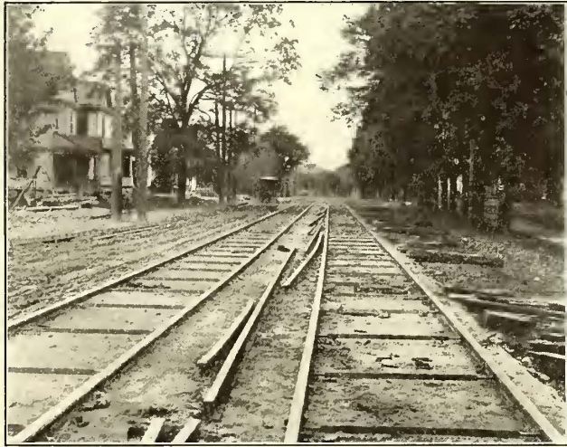
Fig. 22—7-in. T-Rail Construction in South Salina Street, Syracuse
