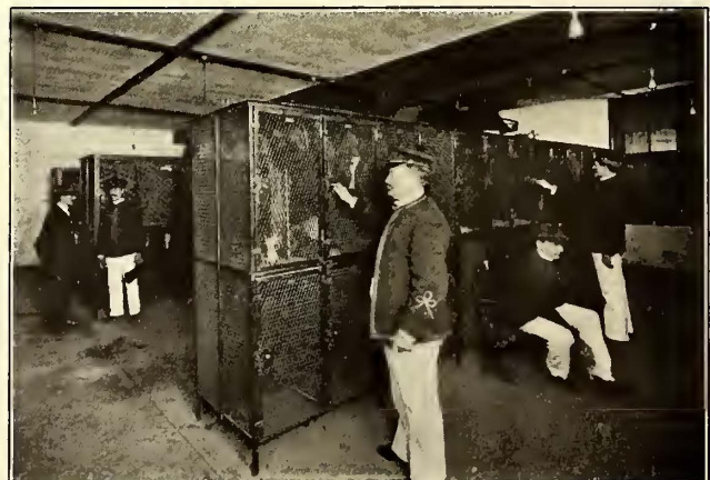
East New York Club House—Locker Room
