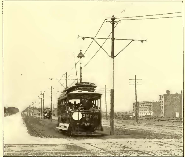
Boston Elevated Railway—Center Pole Bracket Construction on Commonwealth Avenue
