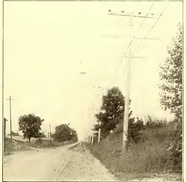
Milwaukee Interurban Lines—High Tension Wire Protection
