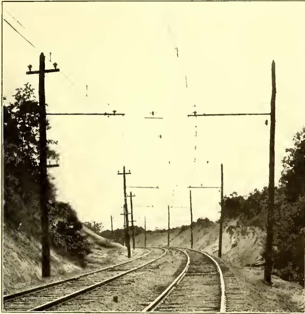
Washington, Baltimore & Annapolis—Backbone Catenary Construction on Curves
