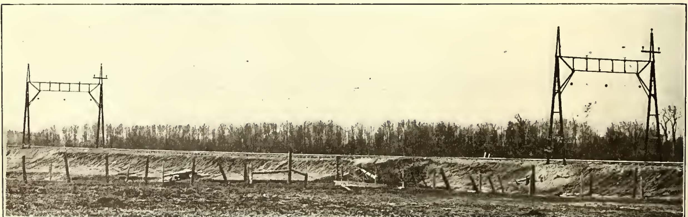
Syracuse, Lake Shore & Northern—Catenary Construction with Steel Bridges
