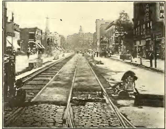
Fig. 24—7-in. T-Rail Construction in South Salina Street, Syracuse
