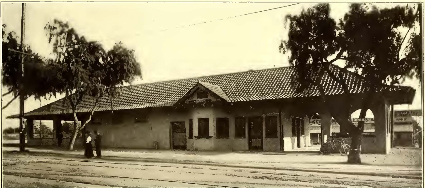
Pacific Electric Railway—Standard Concrete Freight and Passenger Station
