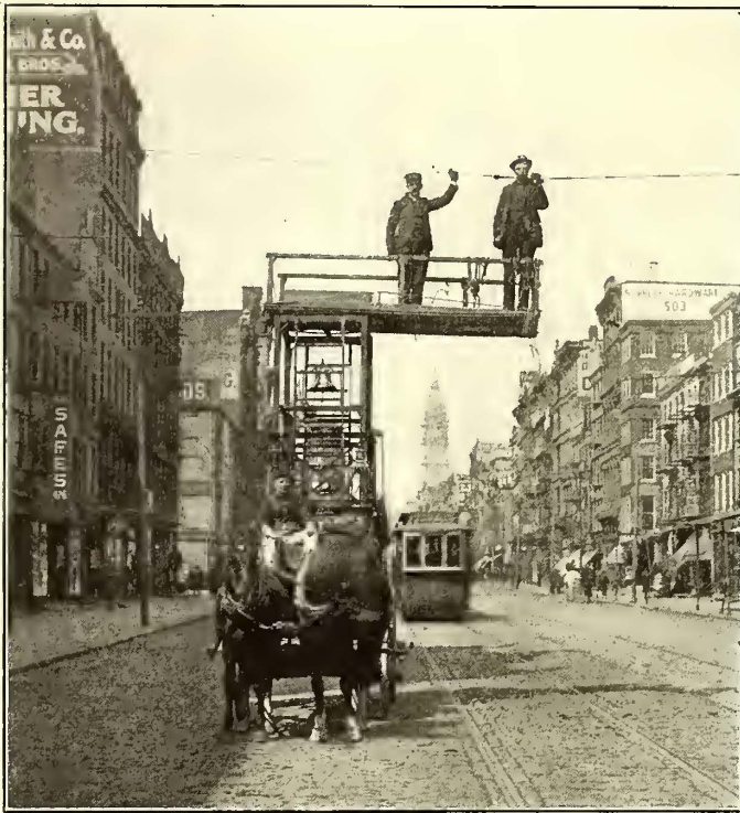
Philadelphia Rapid Transit Company—Extension Tower Wagon
