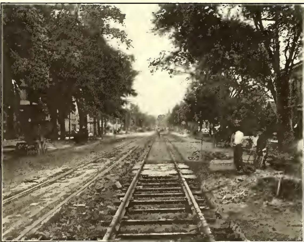
Fig. 23—100-lb. T-Rail Construction in North Salina Street, Syracuse
