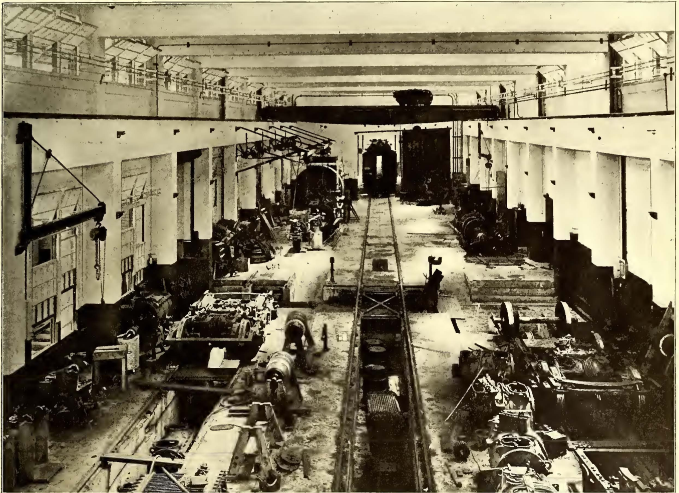
Washington, Baltimore & Annapolis—Interior of Machine Shop
