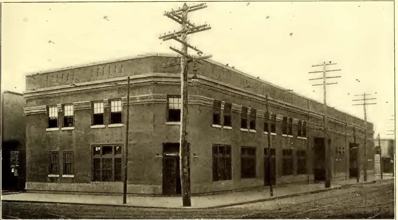
Exterior of Highlandtown Car House, Baltimore
