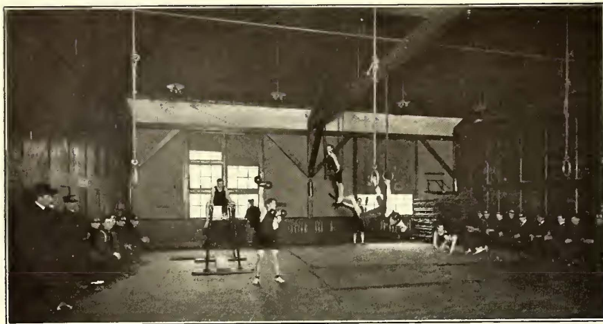
East New York Club House—Gymnasium
