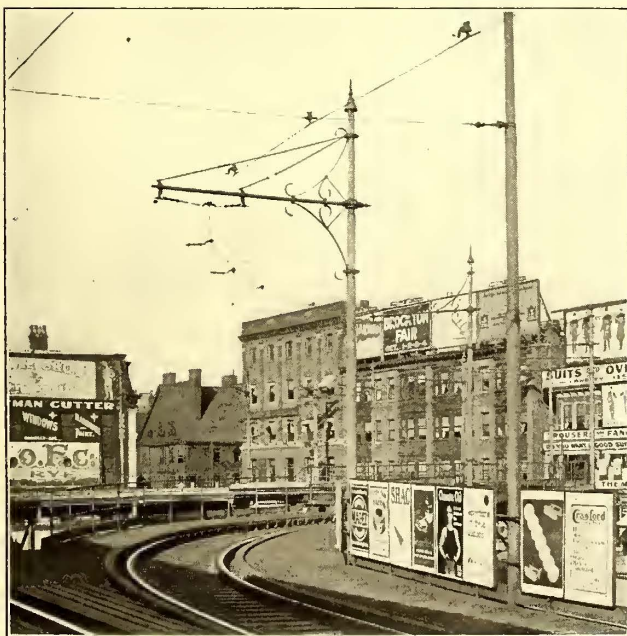
Boston Elevated Railway—Ornamental Bracket Pole Construction at Dudley Street Terminal
