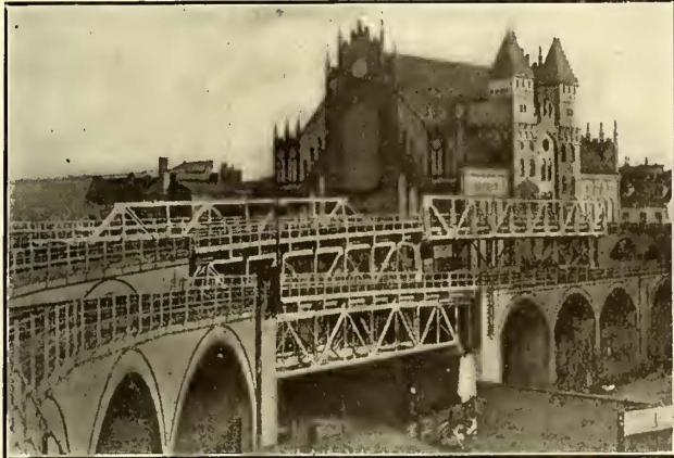
View of Viaduct on Which Accident Occurred
