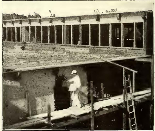
Fig. 16—Method of Applying Cement Plaster to Outside Wall
