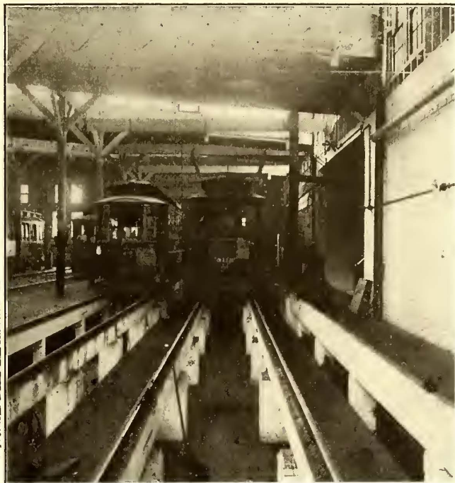
Fig. 28—Drop Floor at Side of Pit
