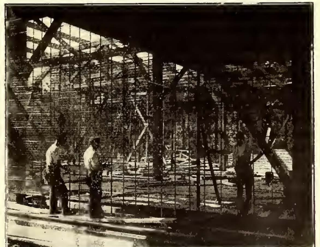
Fig. 38—Plaster Concrete Partition Serving as Fire Curtain
