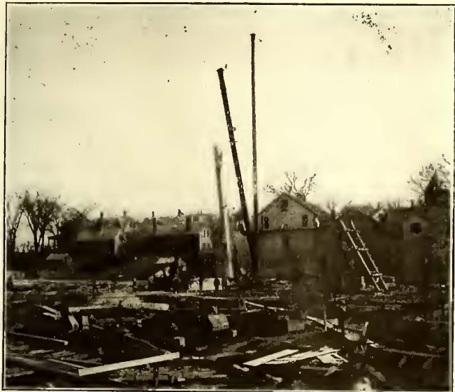
Fig. 21—36-Ft. Concrete Pile Used in the Foundation of Building Shown in Fig. 15
