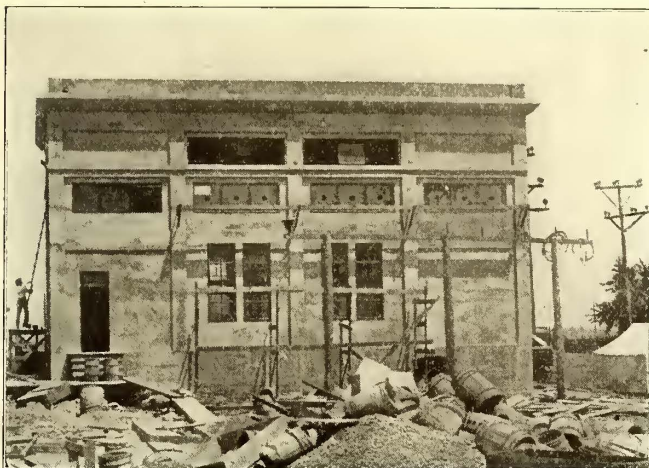
Northern Electric Company—Substation No. 8, Nearing Completion
