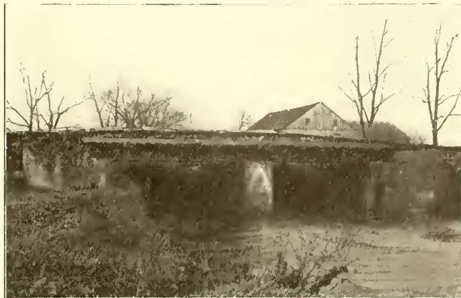
Fig. 4.—Boyertown & Pottstown Railway—Central Pier Bridge over Minister's Creek
