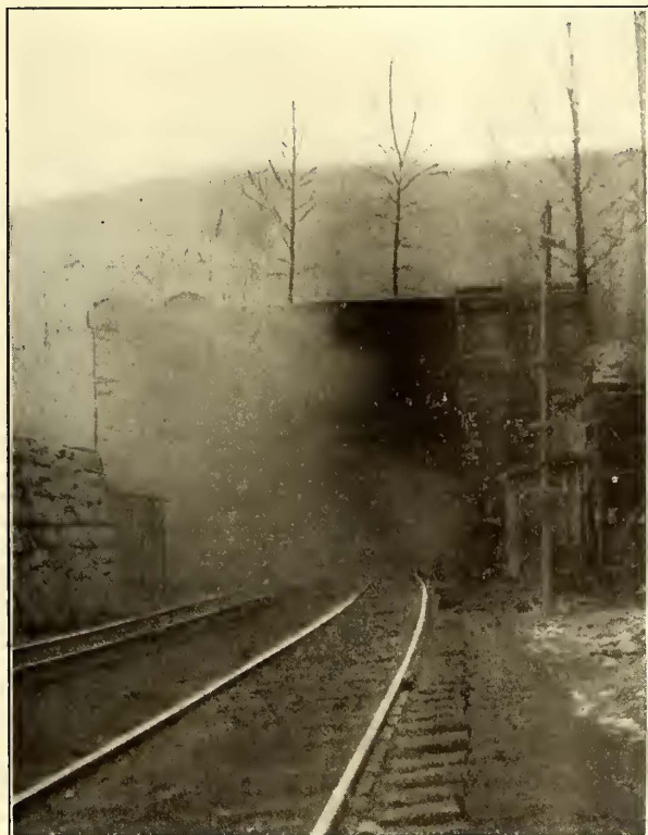
Fig. 4.—Hoosac Tunnel—View of West Portal, Showing Volume of Smoke and Gas Issuing from Tunnel
