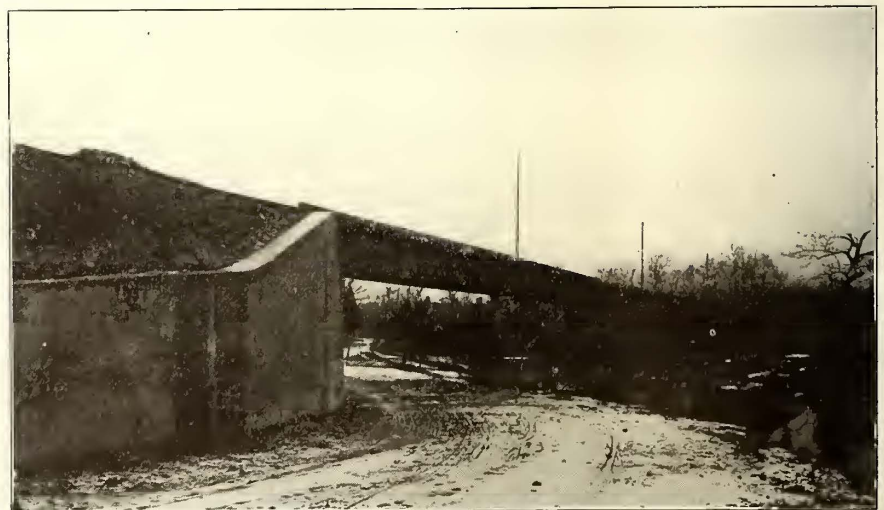
Fig. 2.—Boyertown & Pottstown Railway—Viaduct at Ringing Rocks
