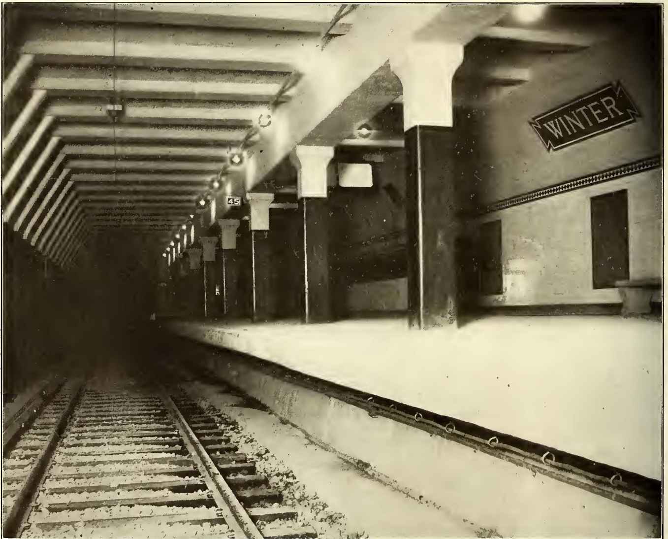
Washington Street Subway—Winter Street Station, Showing Method of Lighting Platforms
