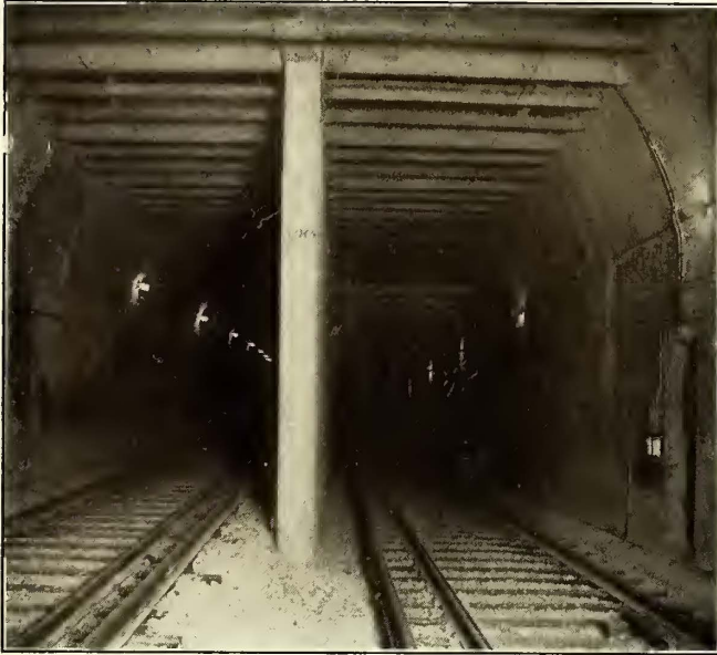
Washington Street Subway—Typical Double-Track Section
