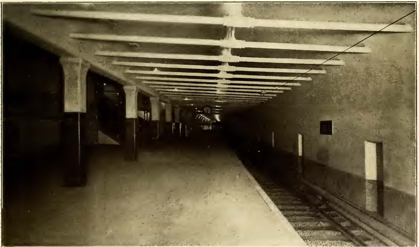
Washington Street Subway—Milk Street Station; Northbound Track Under Platform
