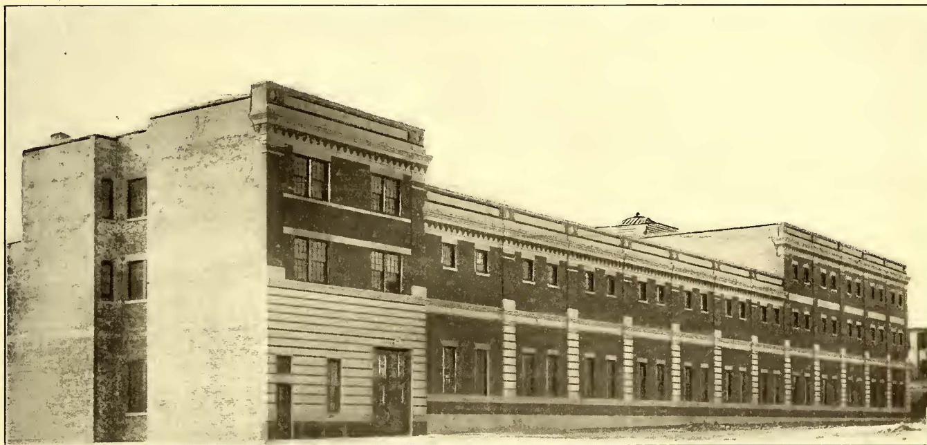
Brooklyn Line and Track Department Headquarters—Elevation Along President Street, with Emergency Building at the Left End
