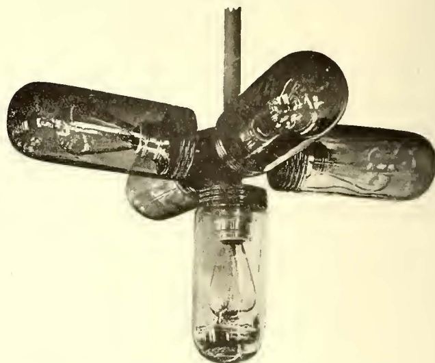
Brooklyn Line and Track Department Headquarters—Five-Lamp Vapor-Proof Cluster
