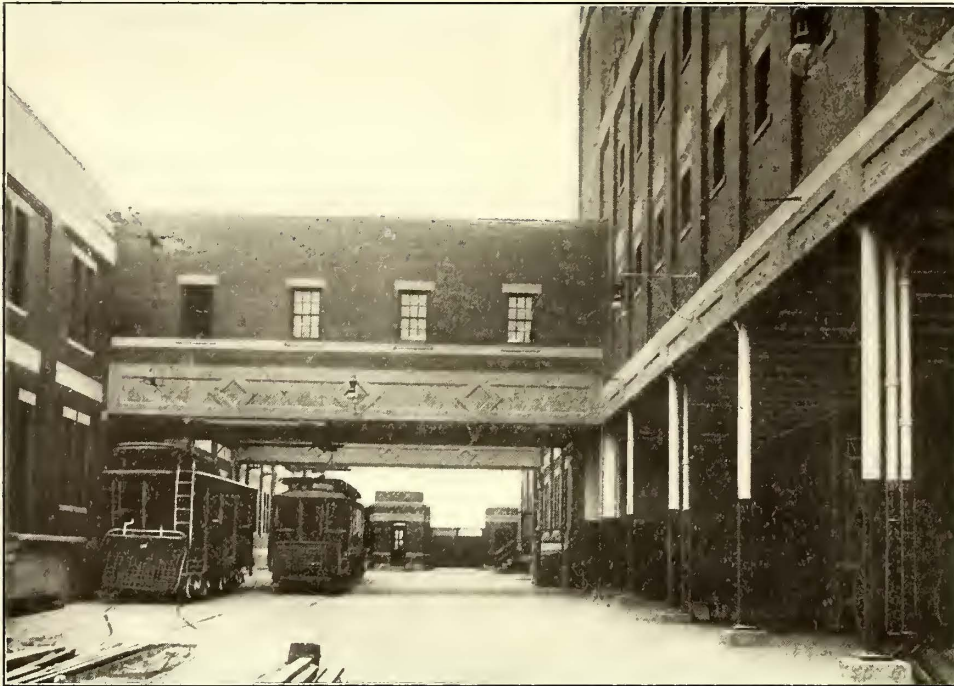
Brooklyn Line and Track Department Headquarters—Looking Along Roadway Toward Watchman's House, with Wagon Storage and Wagon Bridge in the Foreground
