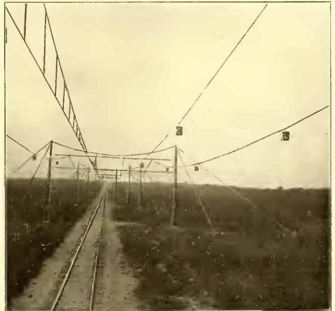
Experimental Trolley Line—Span-Wire Construction for Four Tracks in Section 3
