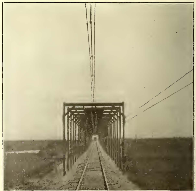
Experimental Trolley Line—Dummy Tunnel with Double Trolley and Secondary Catenary
