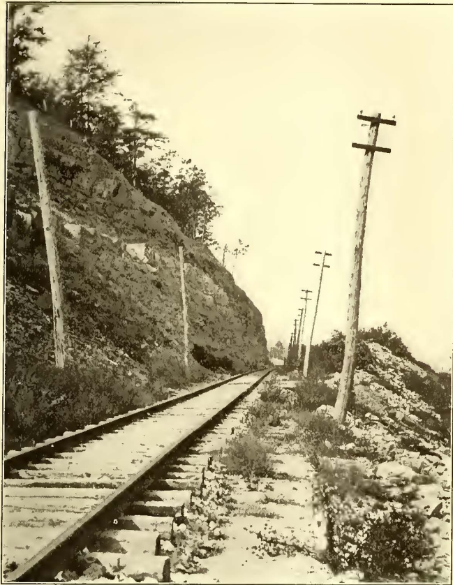
Brantford & Hamilton Electric Railway—Span Suspension for Double Trolley Construction
