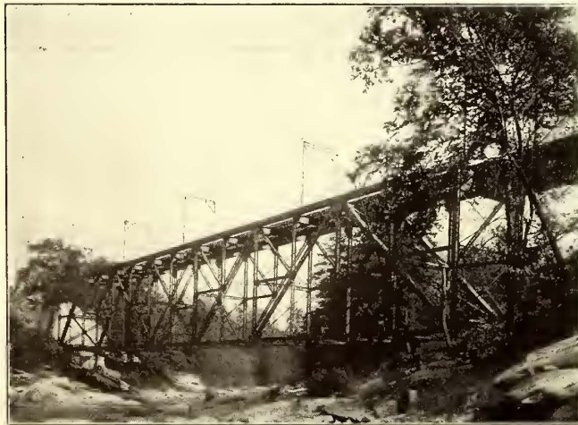
Pittsburg 1200-Volt Line—Buhl Bridge
