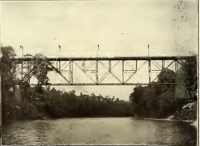
Pittsburg 1200-Volt Line—Grimm Bridge Spanning Connoquenessing River
