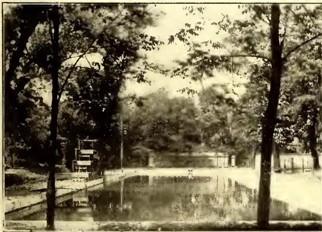
Paxtang Park—The Concrete Swimming Pool and Steps for Diving
