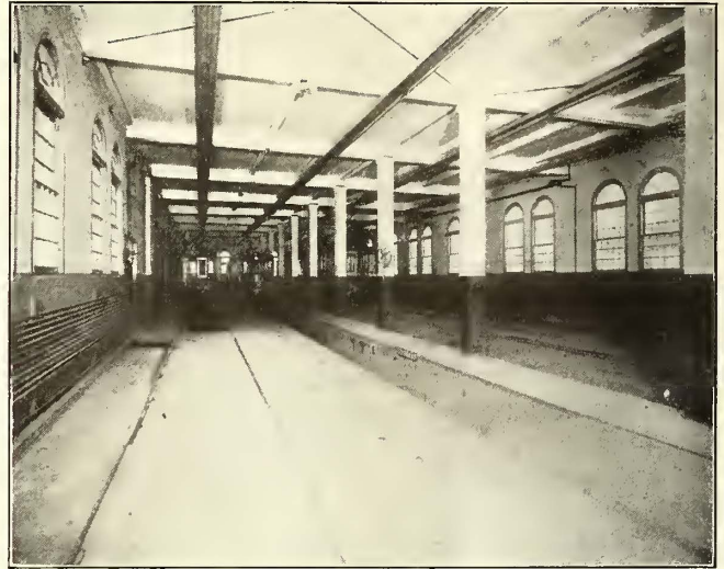
Binghamton Railway—Interior of Utilities Building, Showing General Construction of Pits, Lighting and Heating
