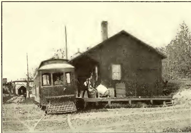
Sheboygan Railway—Typical Freight Station
