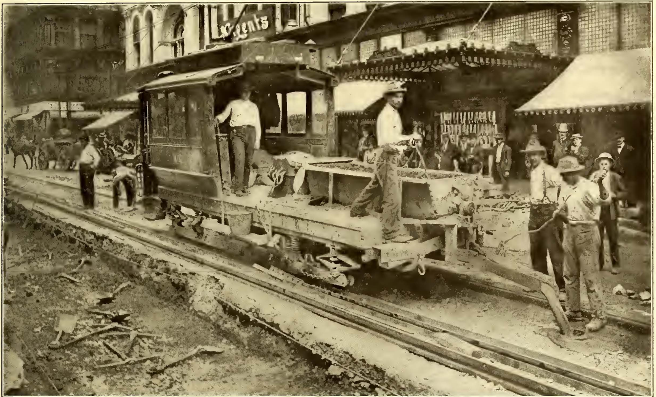
Grout Mixing Machine Built by the United Railways of St. Louis
