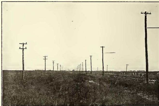
Joplin & Pittsburg—View of 100-ft. Right of Way Showing Double Pole Line
