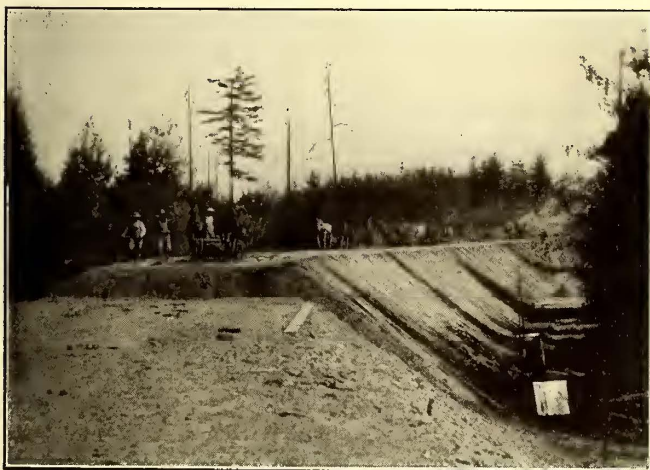
Oregon Railway—Making a High Fill
