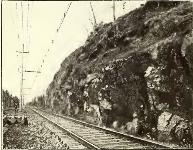
Oregon Railway—View Showing Catenary
