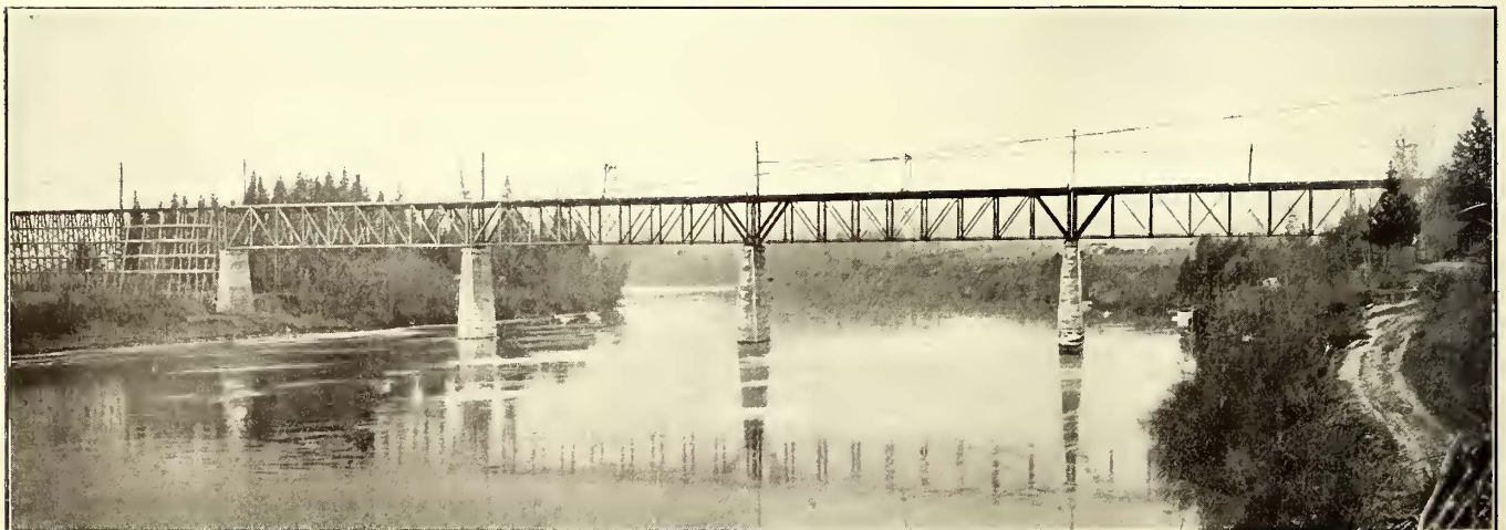
Oregon Electric Railway—Willamette River Bridge
