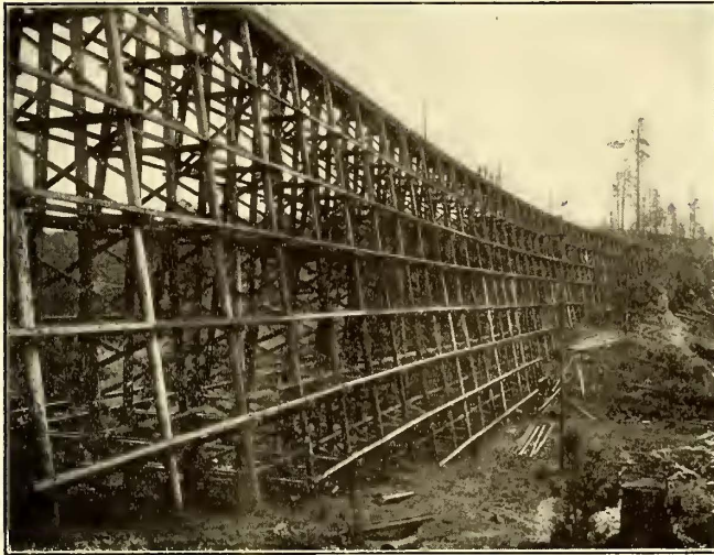
Oregon Railway—Long Trestle
