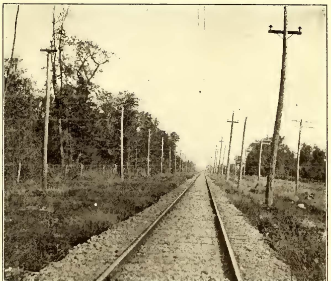
Hamilton Radial Electric Railway—Single-Track Section, Span Type and Double Trolley
