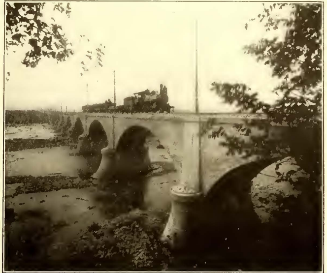
Maumee Bridge—Ballast Train on Bridge
