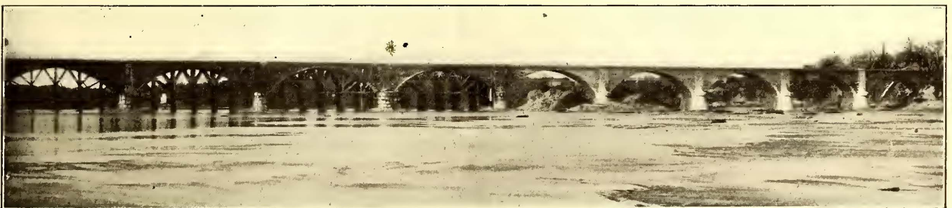
Maumee Bridge—View of Bridge Under Construction
