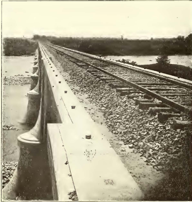
Maumee Bridge—End View, Track Ballasted but Poles Not Erected
