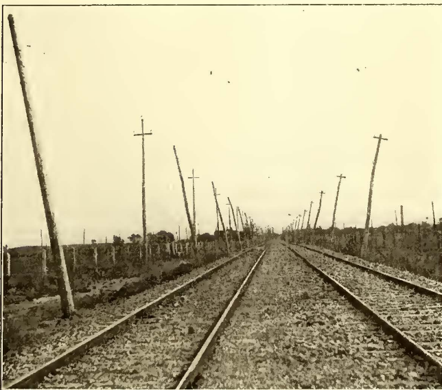
Hamilton Radial Electric Railway—Double-Track Section with Alternating High-Tension Poles on one Side
