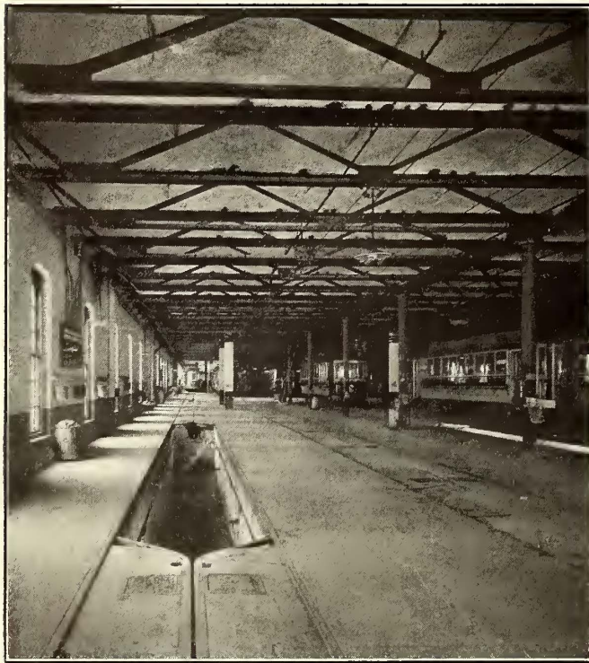
Third Avenue Shops and Car House—Reinforced Ceiling, Concrete Floor and Pit in the Car Inspection Quarters
