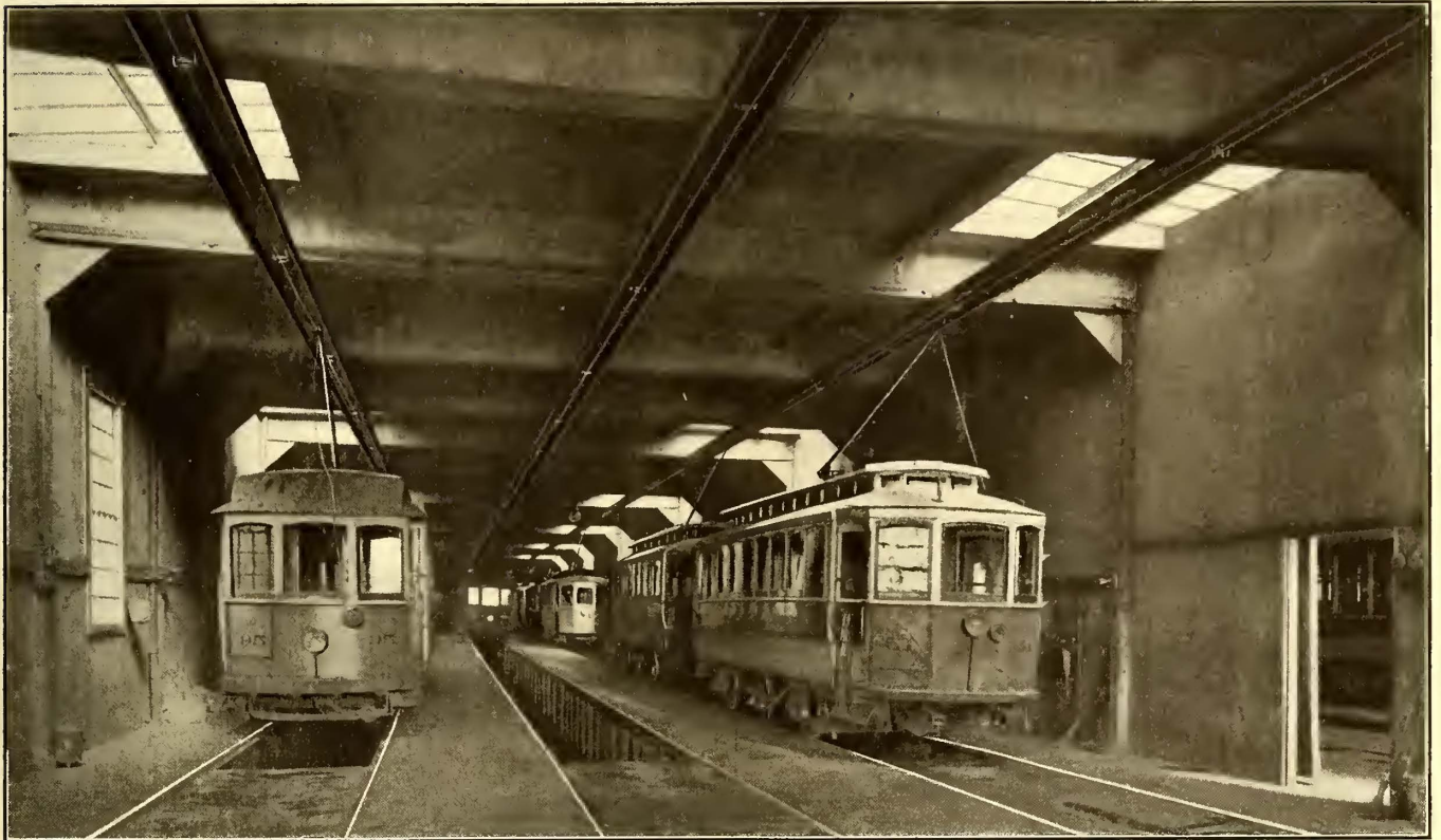
Harrisburg Shops—View of a Bay in the Nearby Car House, Showing the Type of Concrete Construction, Lighting, Pits and Other Features
