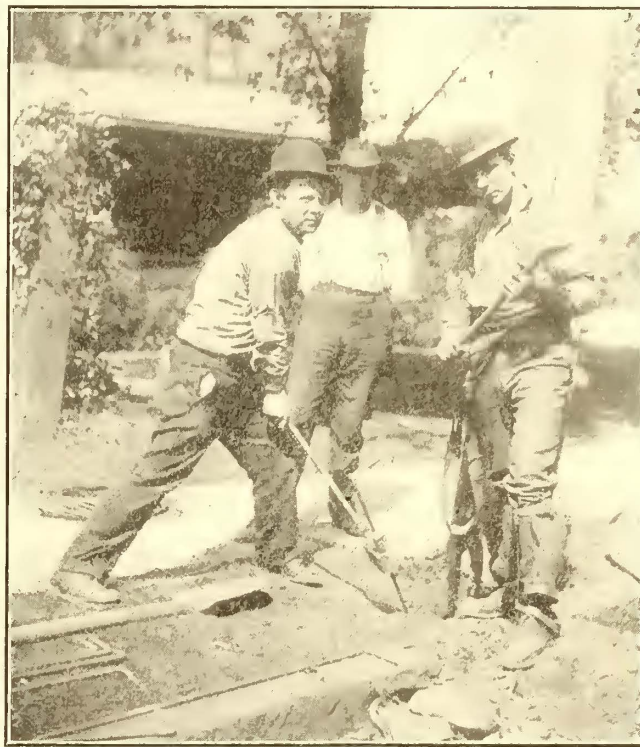
Driving the Reinforcing Rods
