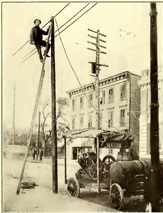
Fig. 4—Pumping Liquid Cement into Pole
