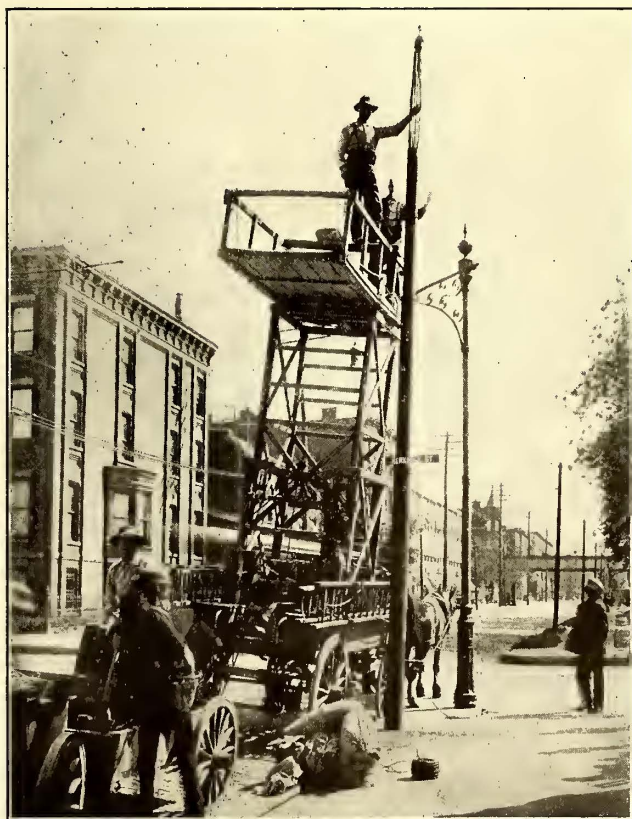
Fig. 3—Slipping the Wires Inside the Pole
