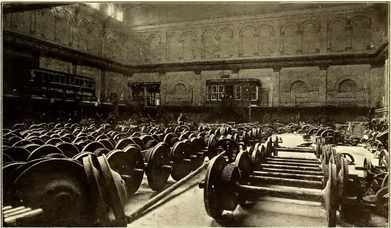
Third Avenue Shops and Car House—View in the New Truck Shop Looking Toward the Car House
