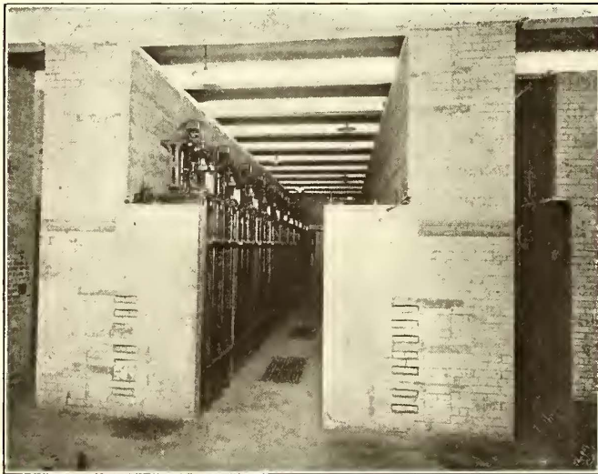
Baltimore Switchboard—Oil-Switch Gallery
