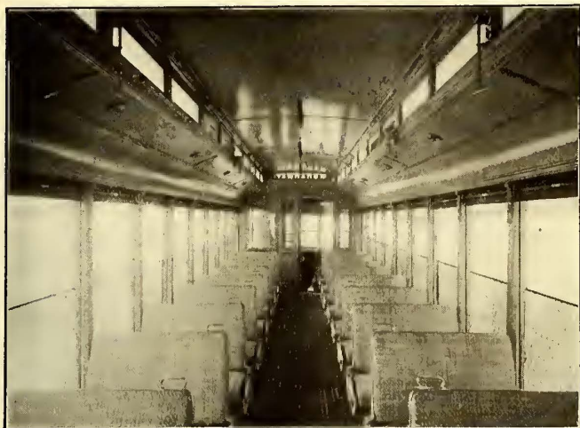
Convertible Pay-As-You-Enter Car—Interior View with Sides Removed
