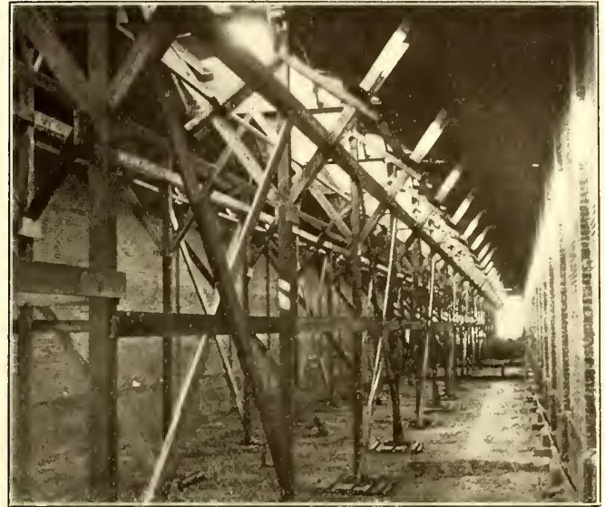
Chicago City Railway Car House—Scaffolding Supporting Roof Slab Forms
