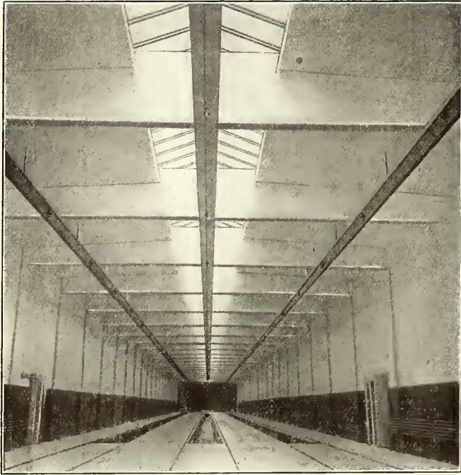
Chicago City Railway Car House—Overhead Lighting in Storage Bay
