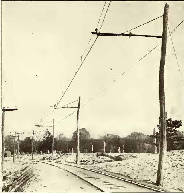
New Canaan Electrification—Construction on Curves Showing Steady Strains
