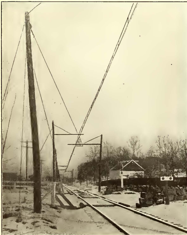
New Canaan Electrification—Overhead Construction with Deflectors at a Siding
