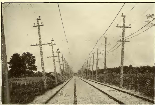
Wooden Pole Line on Rochester, Syracuse & Eastern Railroad
