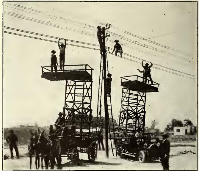
Mexico City Tramways—Mule and Automobile Tower Wagons
