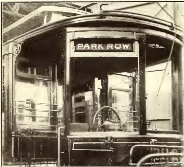
Figs. 4 and 5—Brooklyn Car Lighting—Illuminated Block Sign and Illuminated Curtain Side Sign
