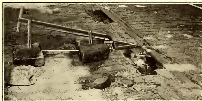
Rail Deflectometer in Service
