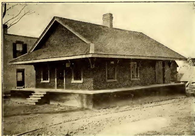
Fig. 3.—Metropolitan Division, Toronto & York Radial Railway—Freight House at North Toronto
