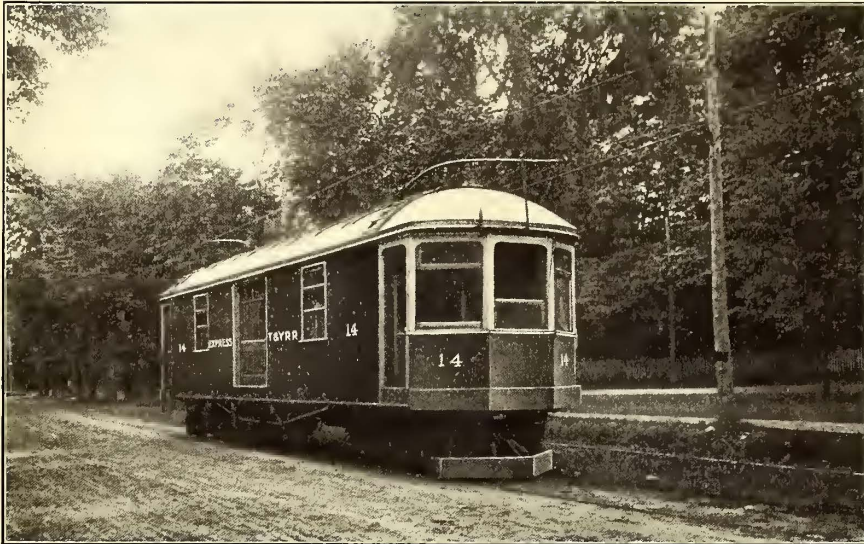
Fig. 1.—Metropolitan Division, Toronto & York Radial Railway—Later Type of Motor Express Car with Side Windows
