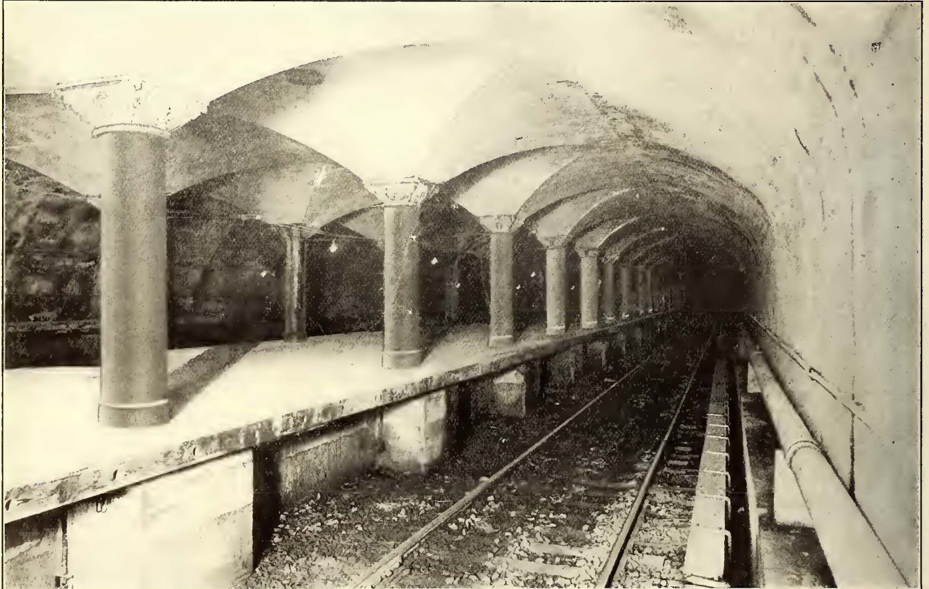
Hudson Terminal—Station Under Erie Railroad Terminal in Jersey City
