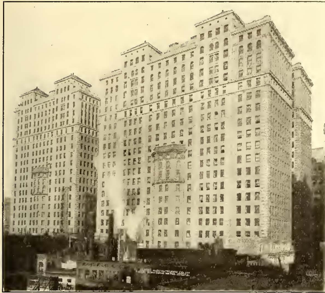
Hudson Terminal—View of Buildings from the River
