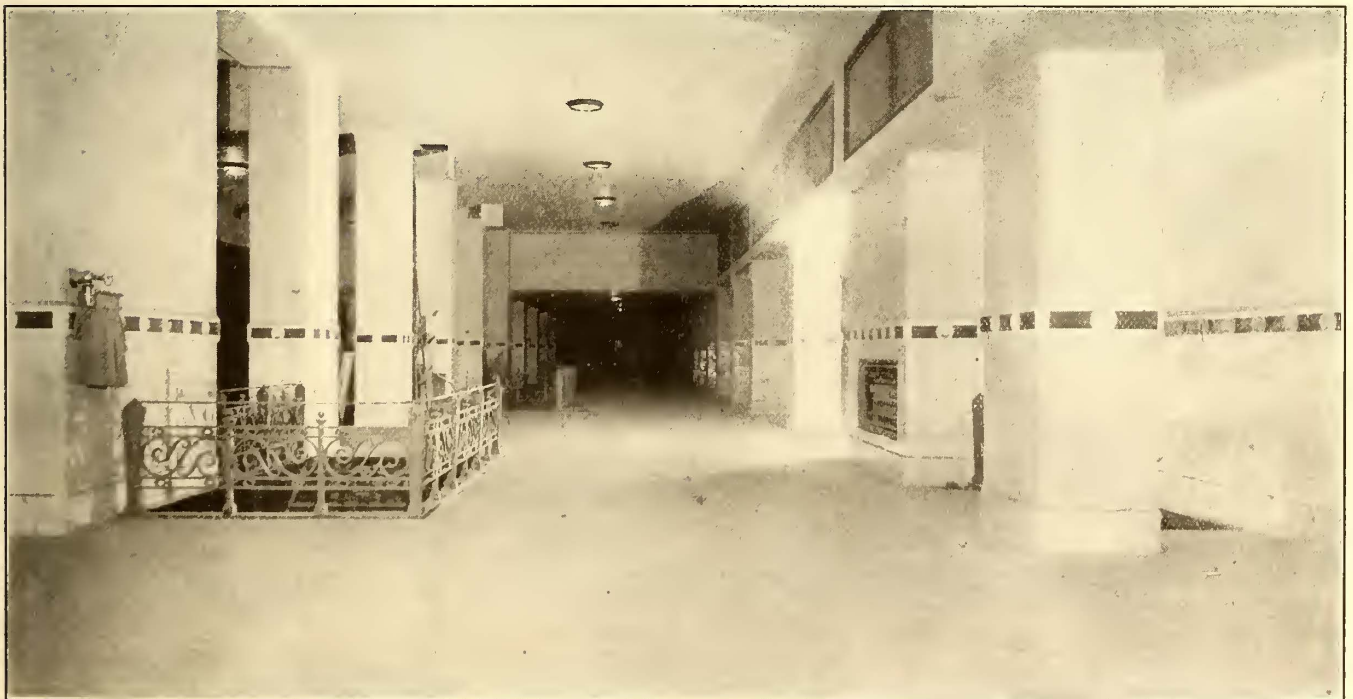
Hudson Terminal—Concourse Level, Showing Stairways Leading to Train Platforms Below
