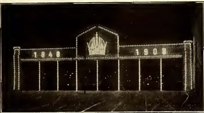
Illumination of Car House
