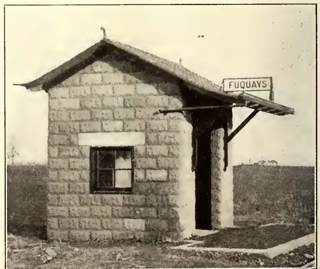
Concrete Block Shelter Station
