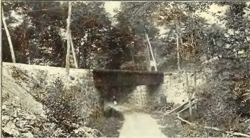
Waterbury Extensions—Steel Girder Bridge Over Highway
