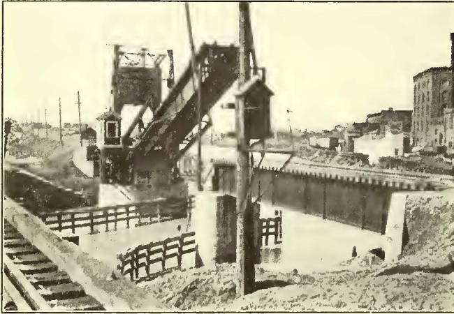
Ohio Electric Railway—Lift Bridge at Toledo, Entrance Open
