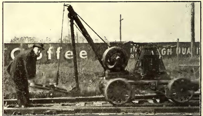
Grinding the Wing Rails of Frogs on the Albany & Hudson Railroad
