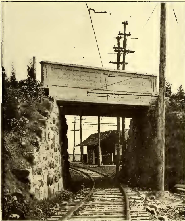
Waterbury Extensions—Reinforced Concrete Slab Bridge, 22-ft. Span, with Middlebury Station in Background
