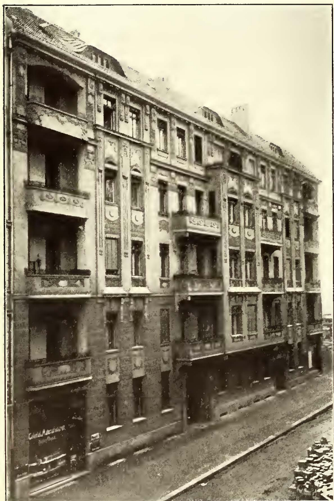
Homes Built for Berlin Railway Men—Front House on Eylauer Street
