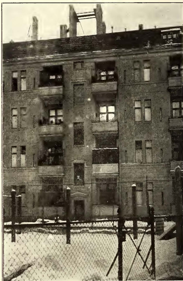
Homes Built for Berlin Railway Men—Courtyard of House in Tegel
