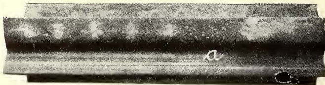
Fig. 6—Rail Corrugation—Head of Rail, Showing Corrugations and Bridging Spots
