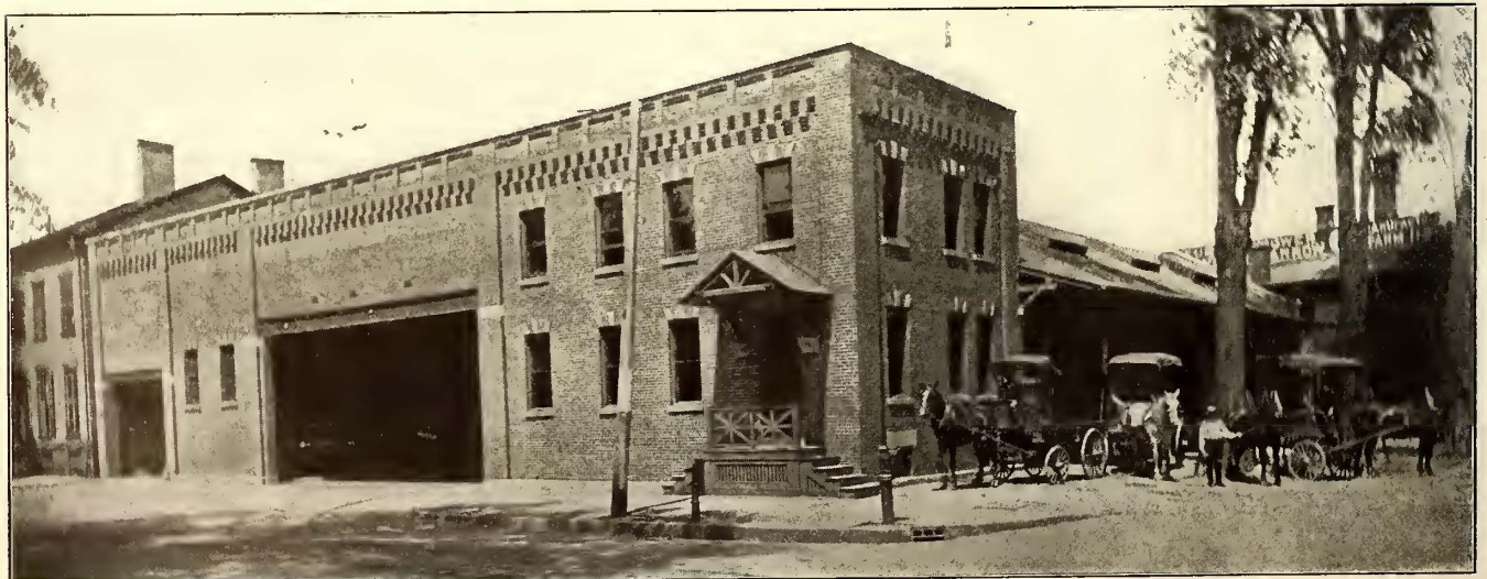
Utica Express and Freight Terminal—Entrance to Warehouse, Tracks in Front, Office at Corner and Wagon Receiving and Delivery Platform at Side
