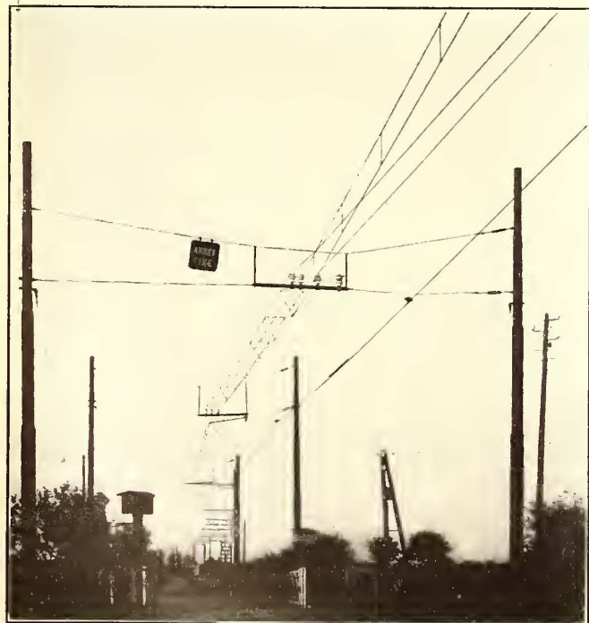
Lyons Single-Phase Tramways—Catenary Construction in the Country
