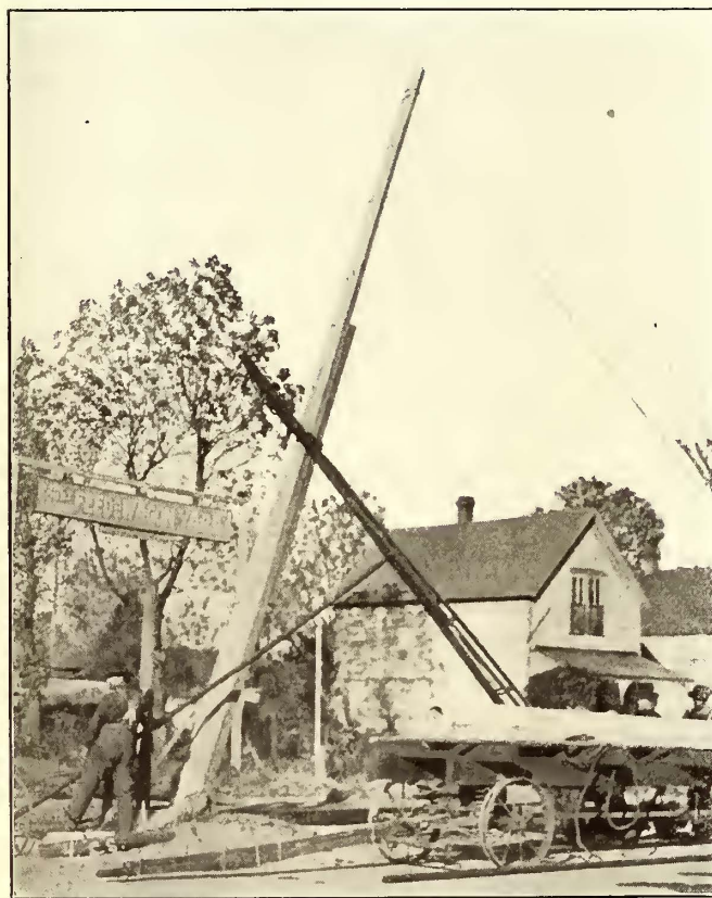
Setting Reinforced Concrete Pole
