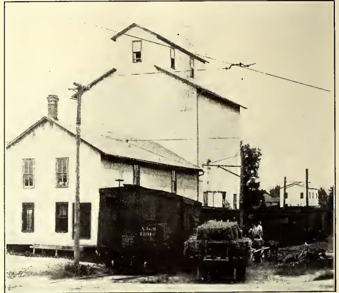
Toledo & Western—Grain Elevator at Pioneer, Ohio
