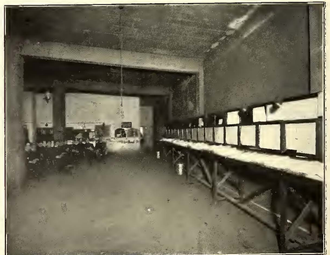
Seattle Electric Company—Division Headquarters, North Seattle
