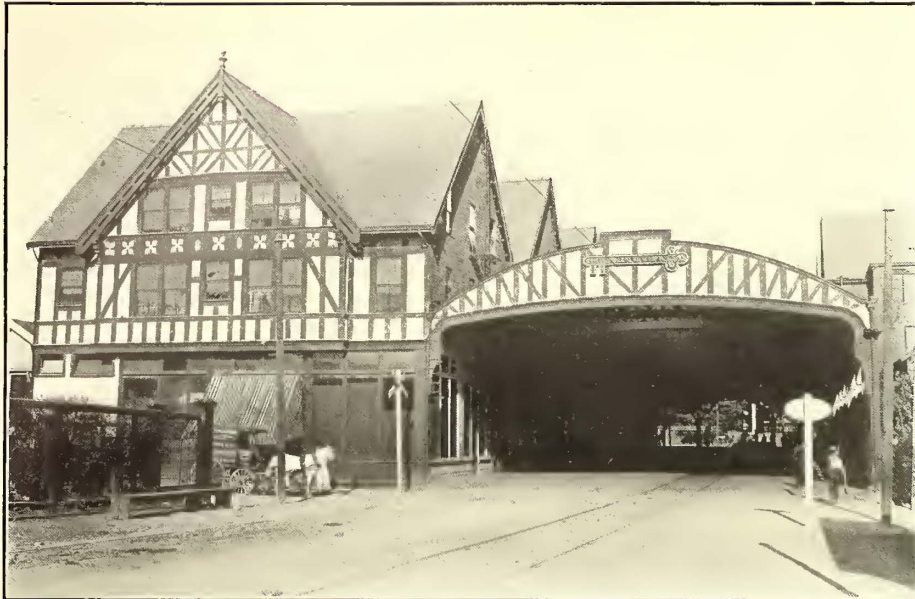
Oakland Electric Railways—Terminal Station and Hotel
