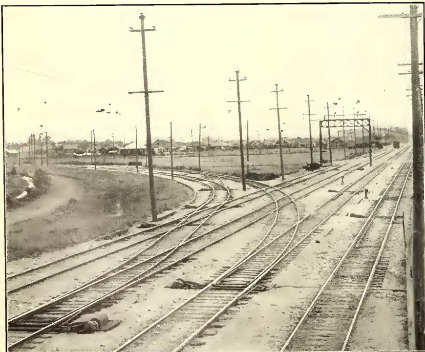
Pacific Electric Railway—Four-Track Entrance to Los Angeles at Branch-Off of Double-Track Line
