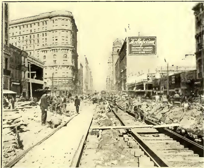
United Railroads of San Francisco—Laying Market Street Track
