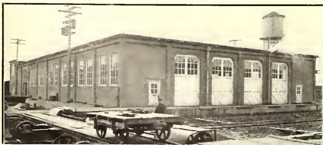
Seattle Electric Company—Erection Shop
