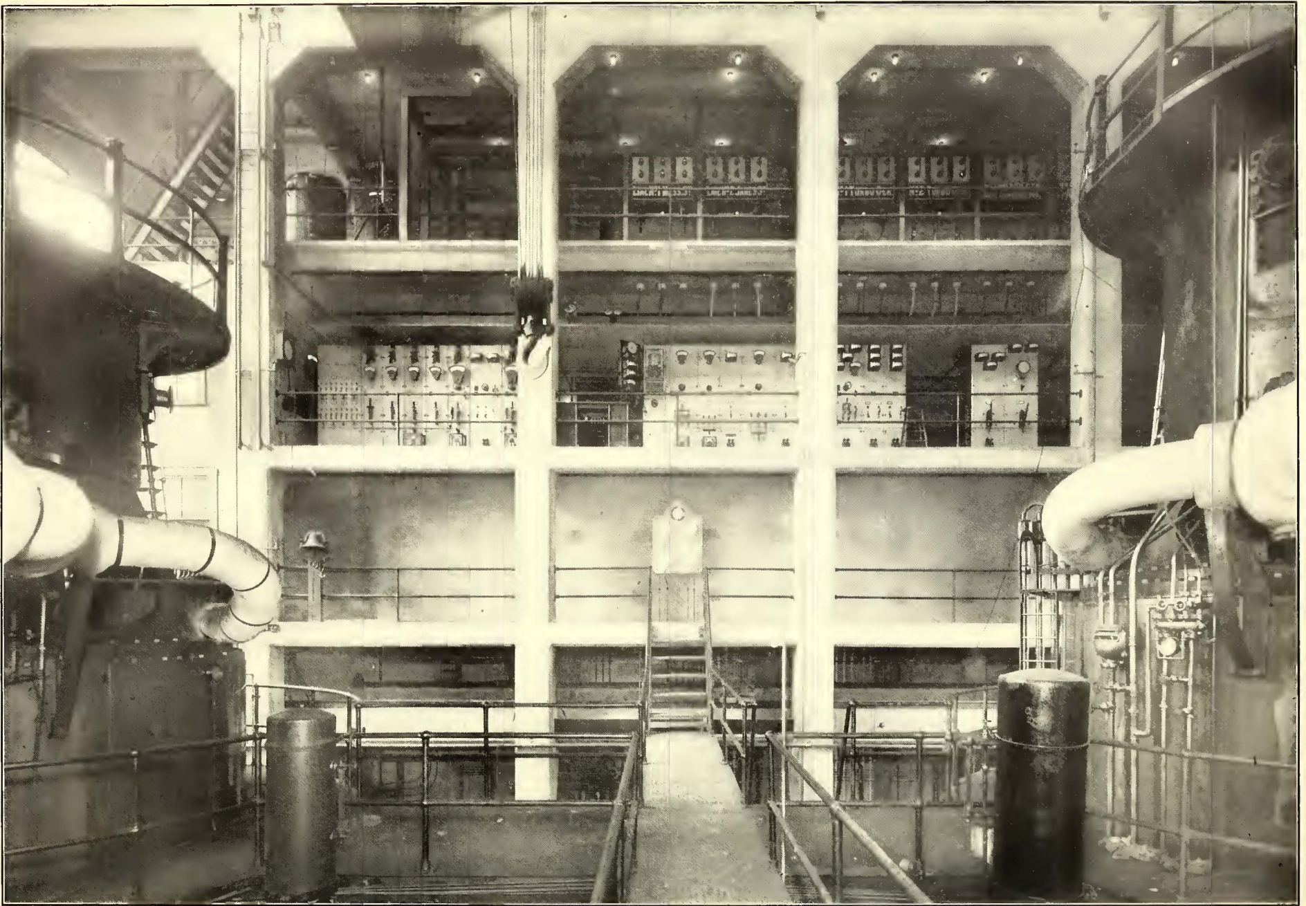
Seattle Electric Company—View of Electrical Galleries in Georgetown Steam Relay Station
