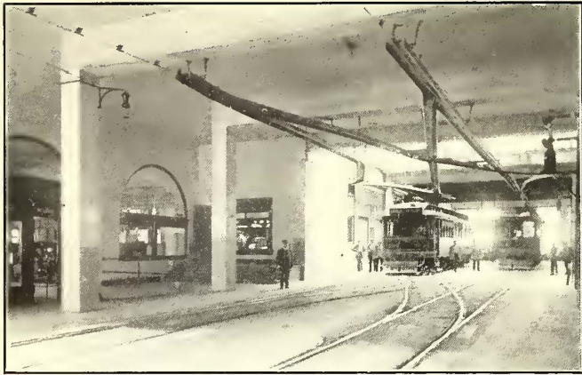
Pacific Electric Railway—First Floor of the Los Angeles Terminal Station
