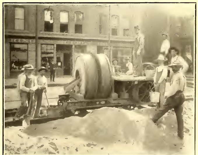
Denver City Tramway—Concrete Mixing Car
