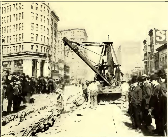
United Railroads of San Francisco—Removing Cable Yokes with Electric Crane
