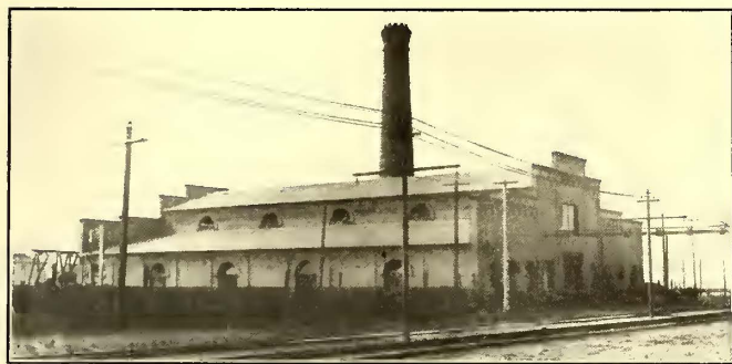
Oakland Electric Railways—Key Route Power Station
