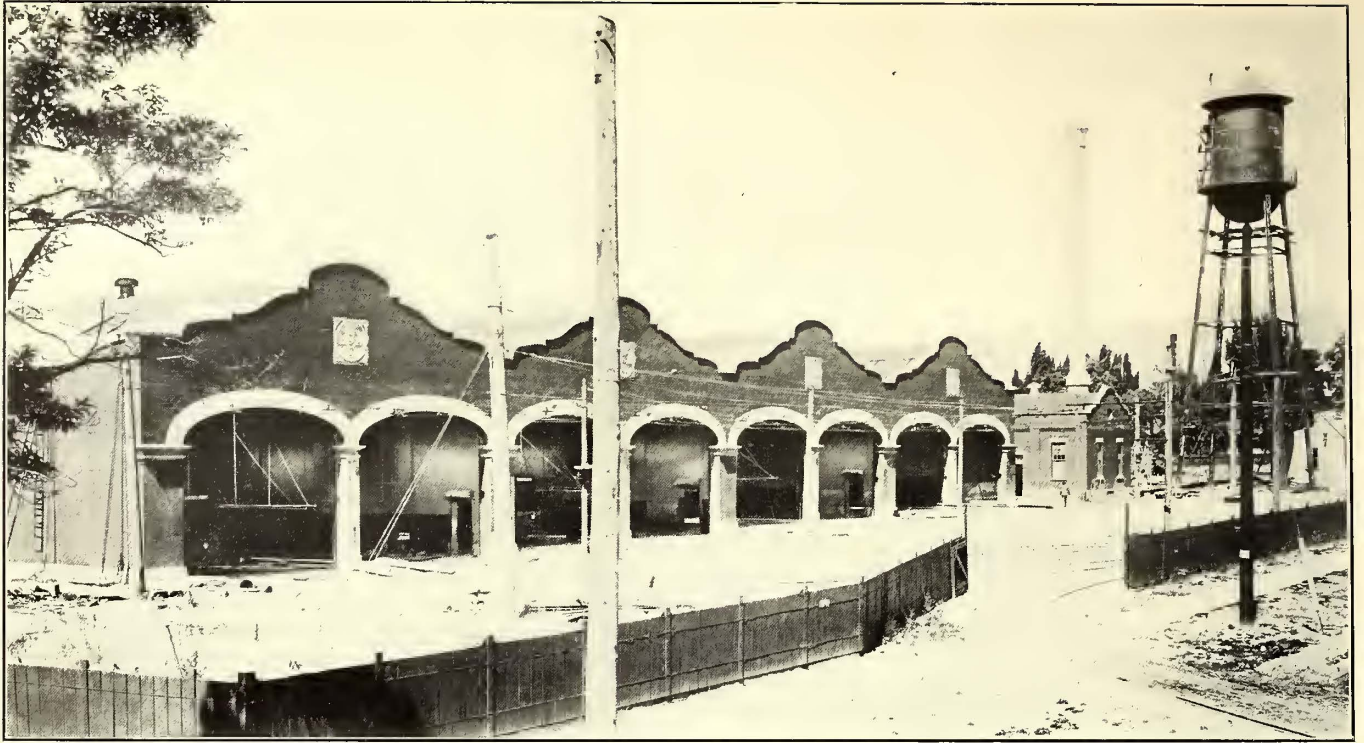
Utah Light & Railway—General View at Front of New Car House, Showing Heating Plant and Elevated Water Tank for Supplying Sprinkler System
