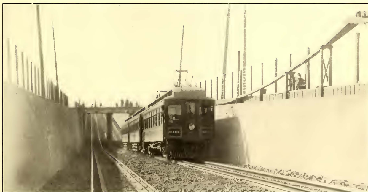
Oakland Electric Railways—Subway Under Southern Pacific Railway
