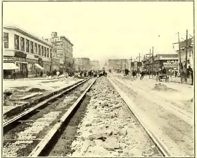
United Railroads of San Francisco—Paving Market Street Track
