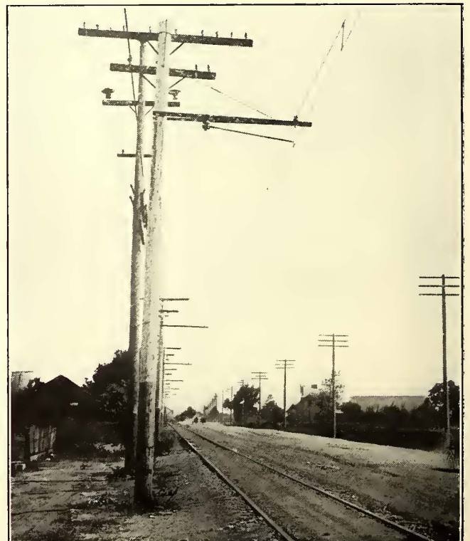
Central California Traction—1200-Volt Catenary Overhead in the City of Stockton
