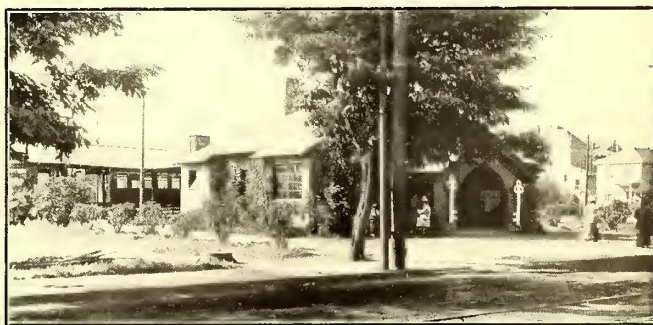
Oakland Electric Railways—Typical Suburban Station
