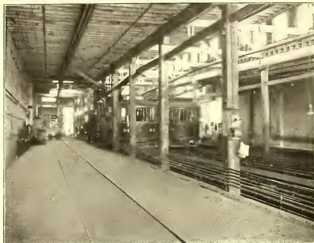
Denver City Tramway—Jacking-up Shop
