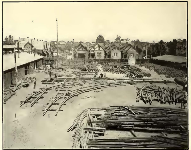
Denver City Tramway—Special Track Work Yard
