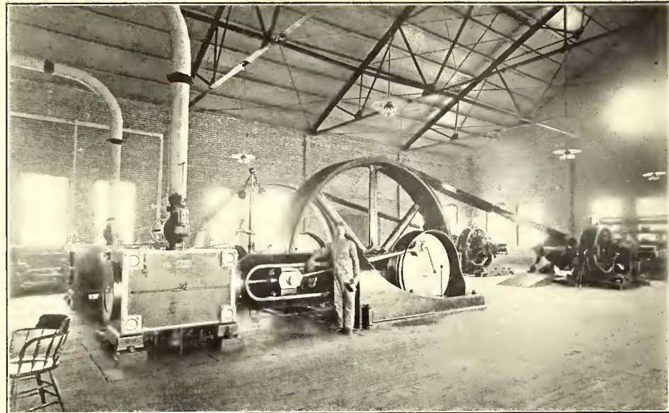
Akron, Bedford & Cleveland—Interior View, Taken in 1899, of Cuyahoga Falls Power House
