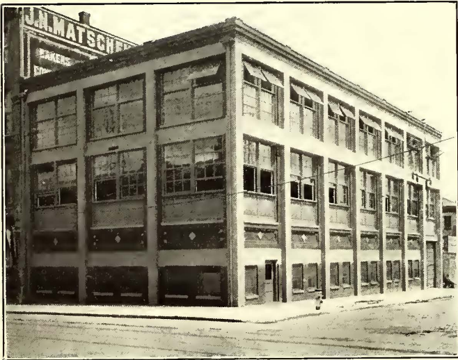
Portland Railway System—South Portland Substation
