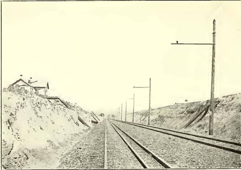
Denver & Interurban Railroad—Electric Track and Double-Gage Steam Track
