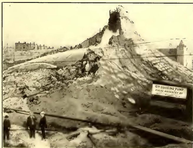
Seattle Electric Company—Cutting Away Denny Hill in 1907
