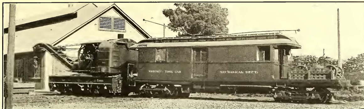
Oakland Electric Railways—Wrecking Tool Car and Crane
