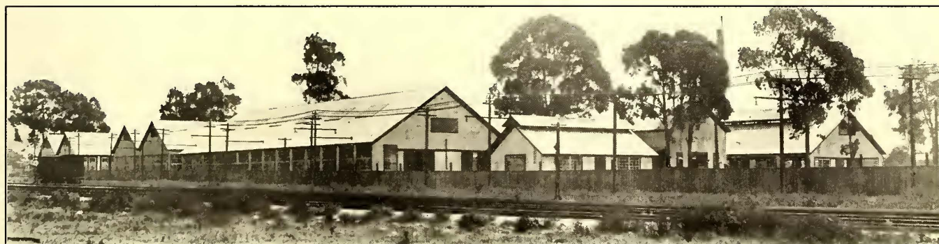
Oakland Electric Railways—Shops of the Oakland Traction Company Located on the Key Route Main Line in Emeryville
