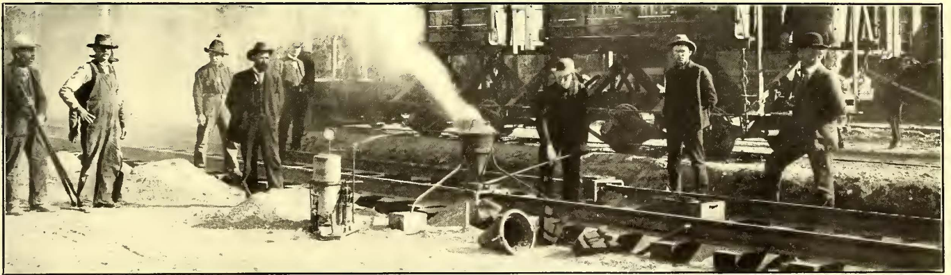
Utah Light & Railway—Welding Track Joints by Thermit Process
