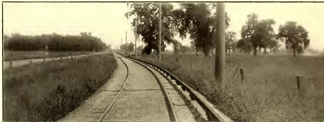
Northern Electric Railway—Third-Rail Track
