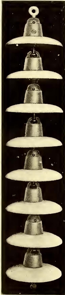
High-Tension Porcelain Insulator
