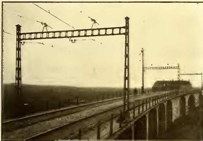
Scheveningen Single-Phase Railway—Viaduct in the Outlying Portion of Rotterdam
