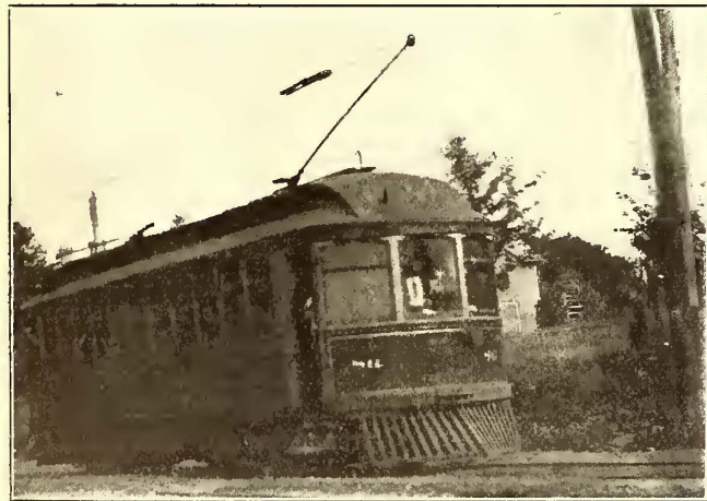
Automatic Signal at Switch in Hubbard, Ohio
