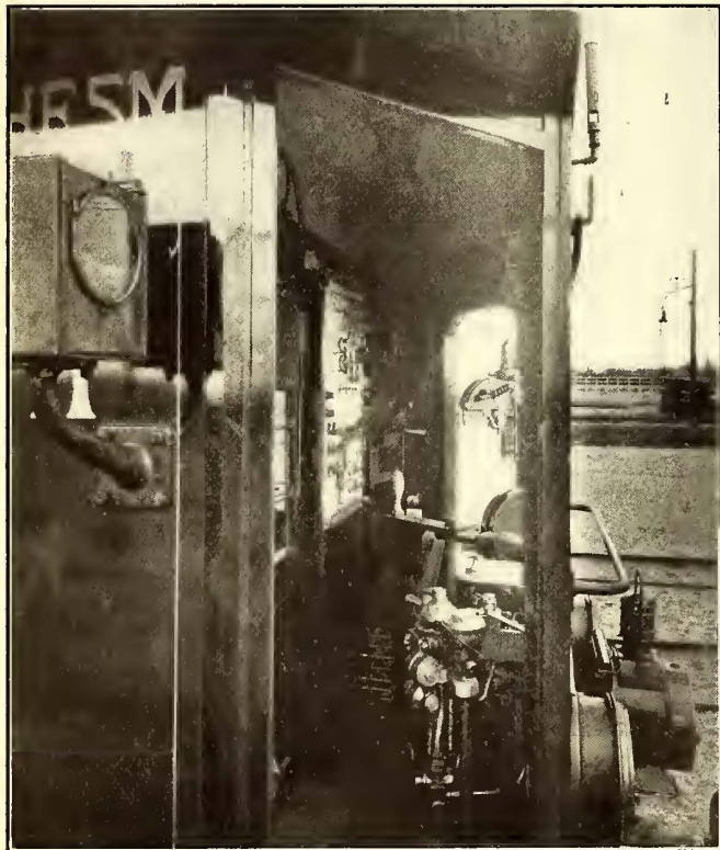
Scheveningen Single-Phase Railway—View in Motorman's Cab
