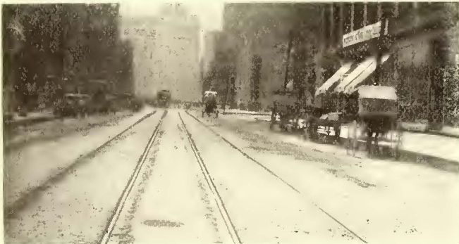
Way Matters—One of the Most Congested Streets in Milwaukee with Pavement Eight Years Old.
