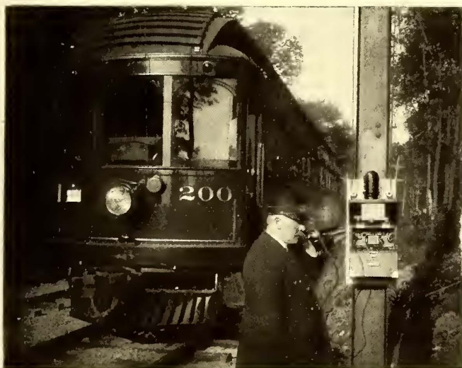
Fig. 1—Portable Telephone Set Connected to Jack Box
