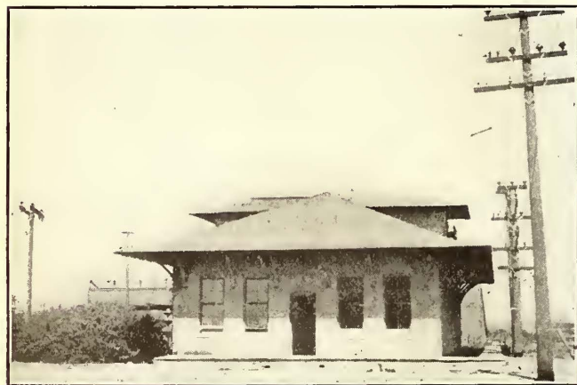
Los Angeles Pacific Company—Substation at Plaza del Rey struction of the completed buildings, and has not yet been replaced with the permanent layout. This will probably be done in the near future.
