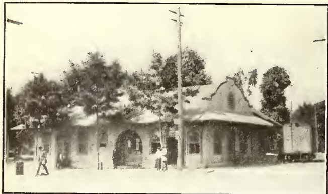
Los Angeles Pacific Company—Passenger and Freight Depot at Sawtelle
