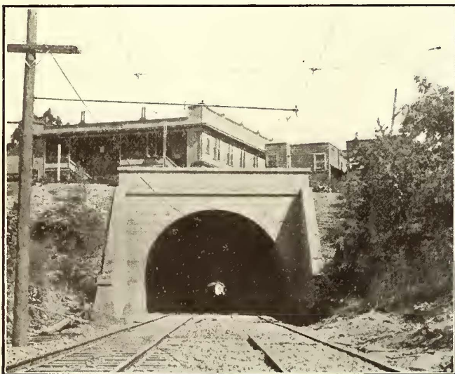
Los Angeles Pacific Company—South Portal, Tunnel No. 2
