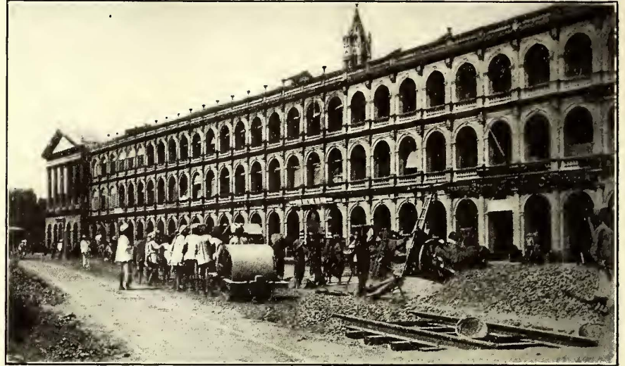
Bombay Tramways—Rolling Ballast with Hand Roller
