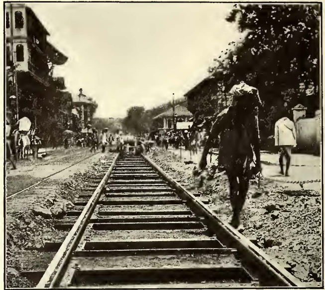
Bombay Tramways—Completed Track Ready for Paving
