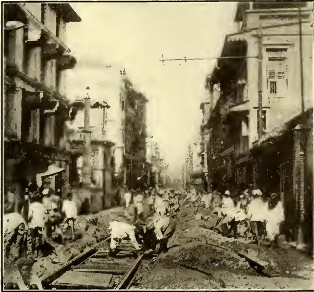
Bombay Tramways—Single Track Bracket Pole Construction in a Narrow Street
