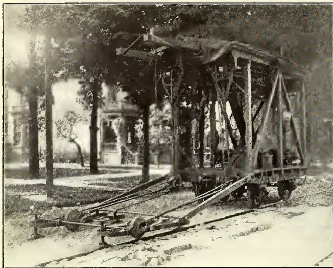
Detroit United Railway—Rail Joint Grinder
