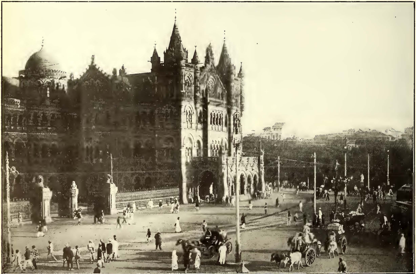
Bombay Tramways—Bori Bunder Junction in Front of the Victoria Terminal Station
