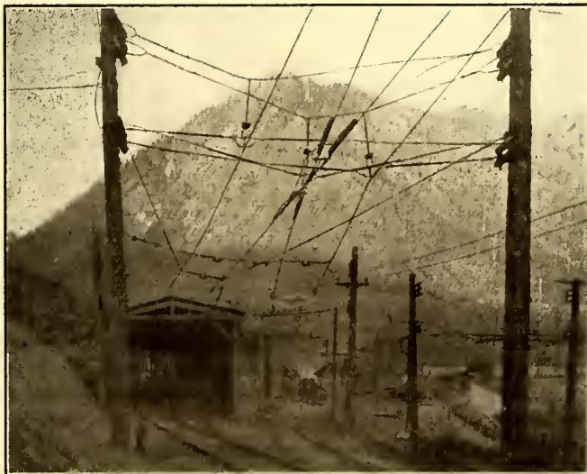
Great Northern Electric System—Overhead Construction Above Switch Point in Wellington Yard
