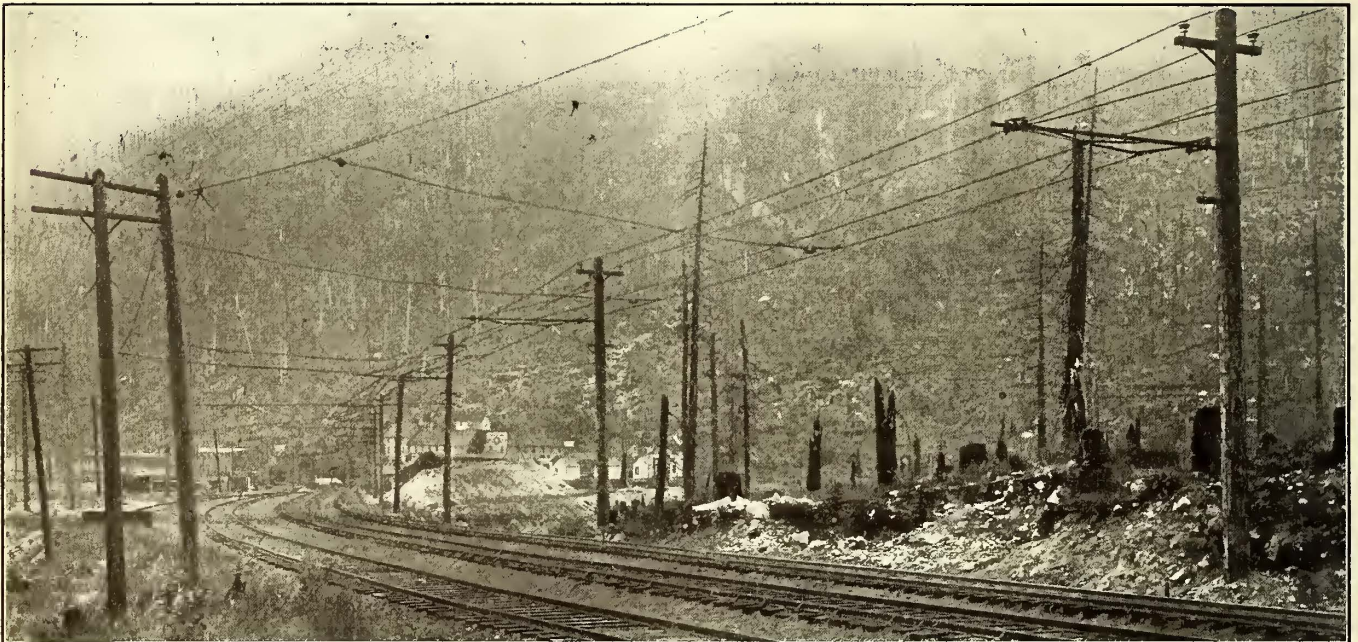
Great Northern Electric System—Cascade Yard Showing Bracket Construction on Curve
