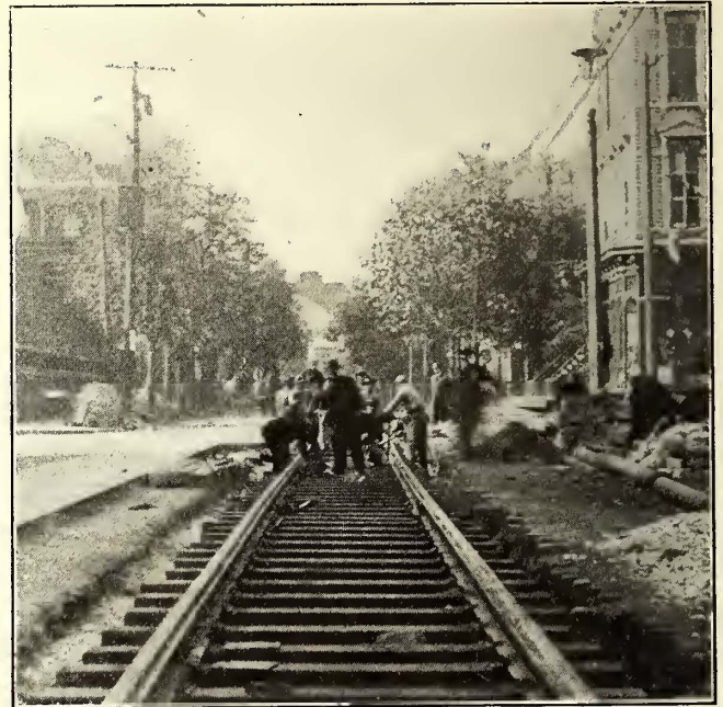
Coney Island & Brooklyn Track Improvements—Tie-Plate Construction at DeKalb and Evergreen Avenues
