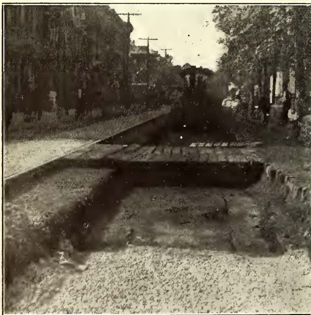
Coney Island & Brooklyn Track Improvements—Roller Use on Sub-Grade
