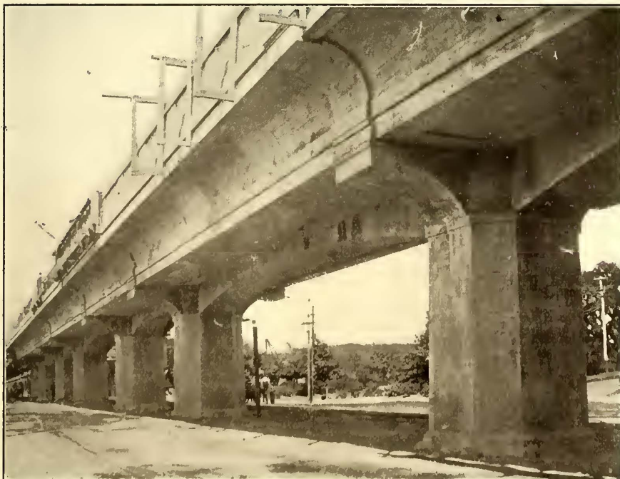
Boston Elevated Extensions—Forest Hills Structure Nearing Completion
