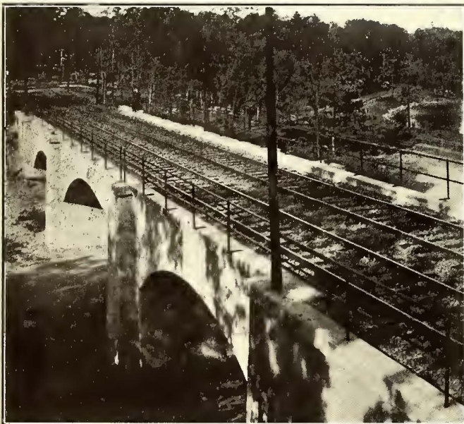
Boston Elevated Extensions—Brooks Road Bridge at Middlesex Fells
