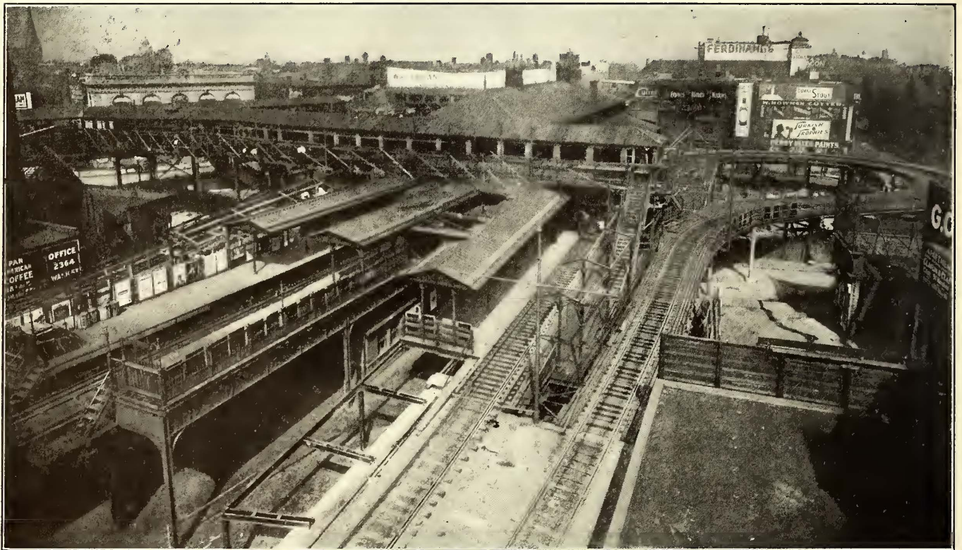
Boston Elevated Extensions—Changes under Way at the Dudley Street Station
