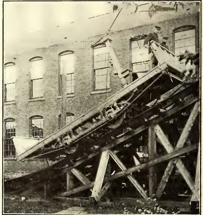
Truck Equipped with Magnetic Car Wheels on Heavy Grade
