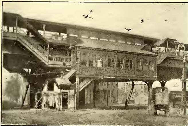
Boston Elevated Extensions—Egleston Square Station Built Largely of Reinforced Concrete
