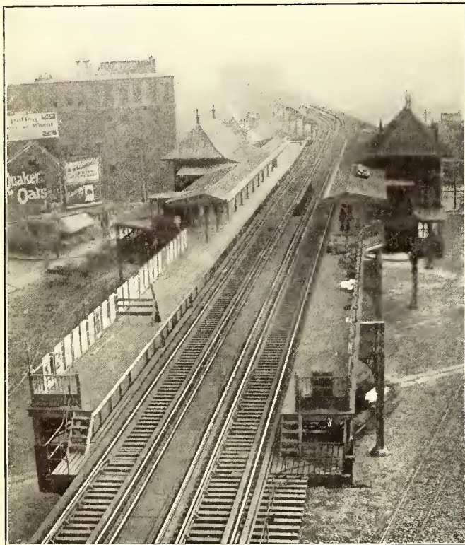
Boston Elevated Extensions—Remodeled Station at City Square
