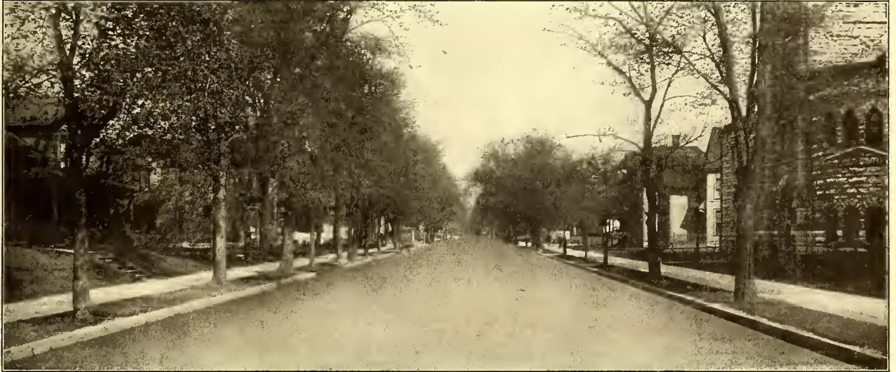
Twelfth Street South, Minneapolis. Wood Block Pavement Filled with Barrett's Paving Pitch
