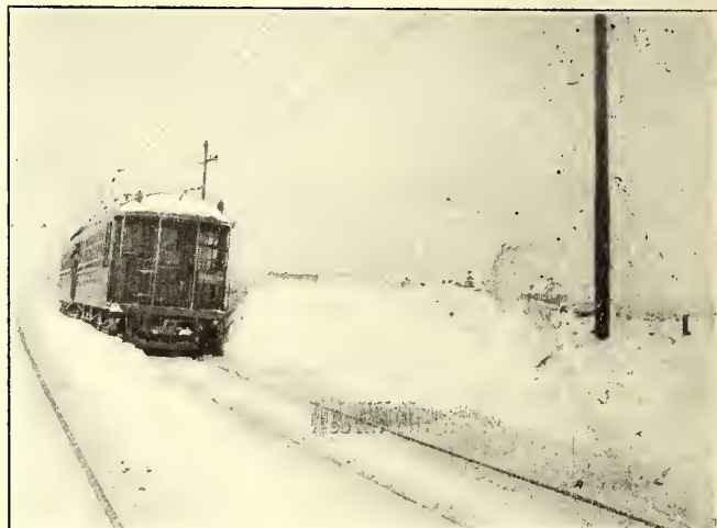
View Along West End Line After Opening for Service
