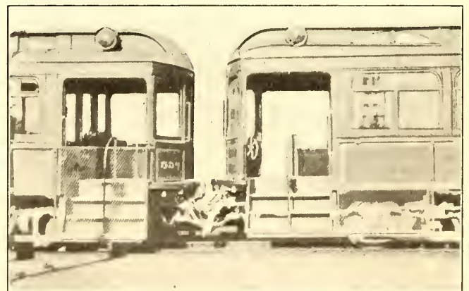
Key Route Cars—Sliding Platform Gates
