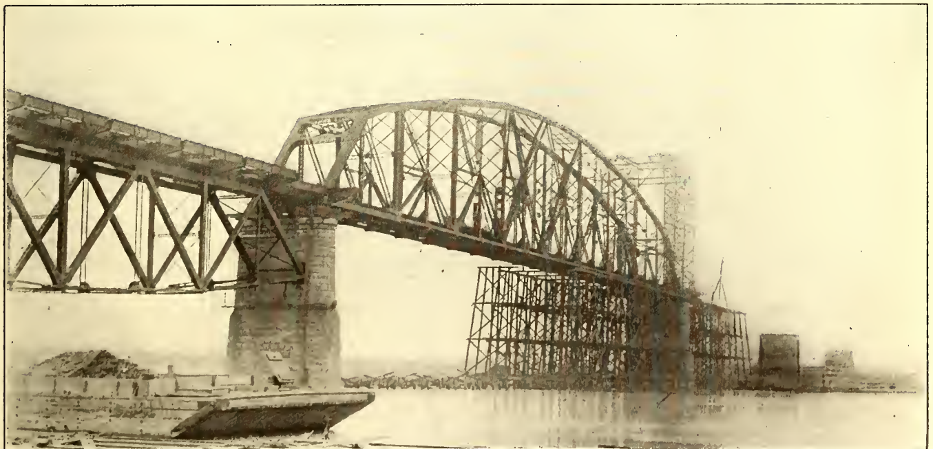
Illinois Traction System—McKinley Bridge over the Mississippi River, Nearing Completion
