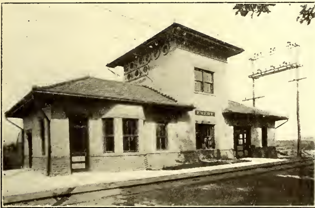
Illinois Traction System—New Standard Passenger Depot and Substation
